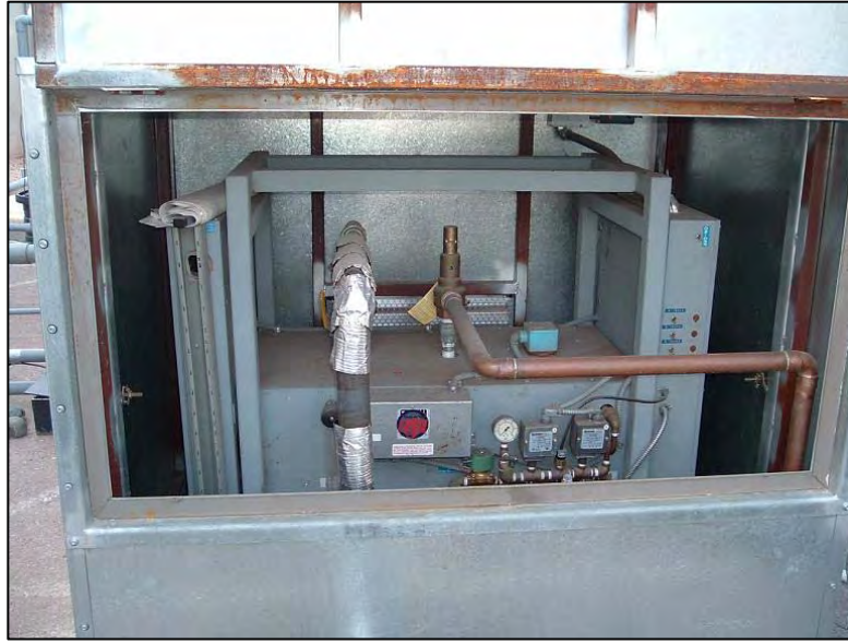
Figure 18. Electric steam boiler in its enclosure.
