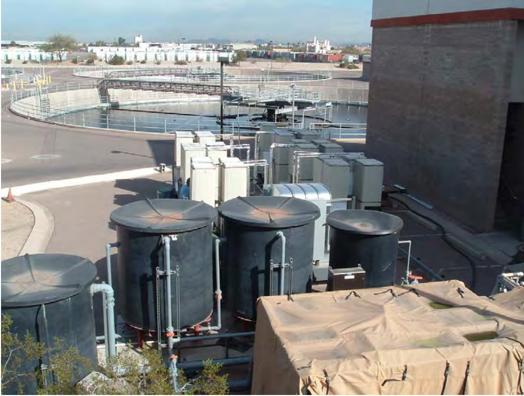
Figure 7. Towers installed at pilot site with generator, tanks, and tactical water purification system.
