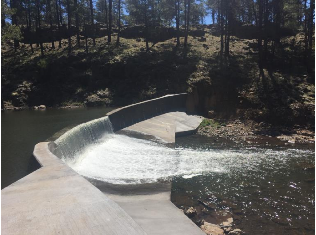
Figure 5. West Fork Black River fish barrier.
