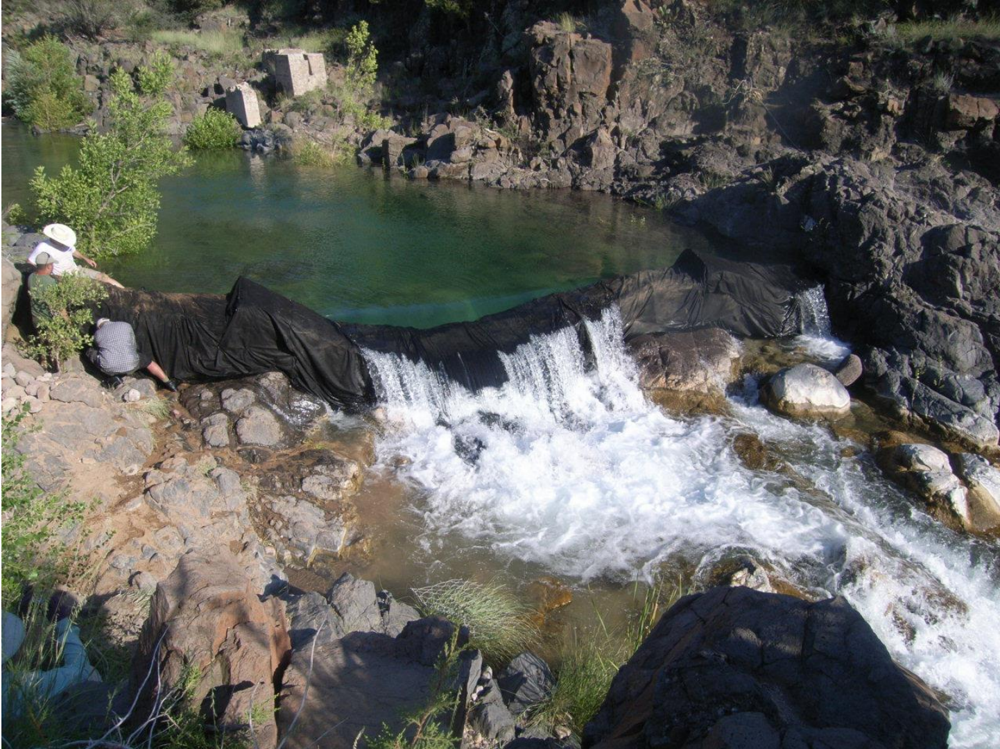
Figure 7. Completed temporary fish barrier at Fossil Creek.
