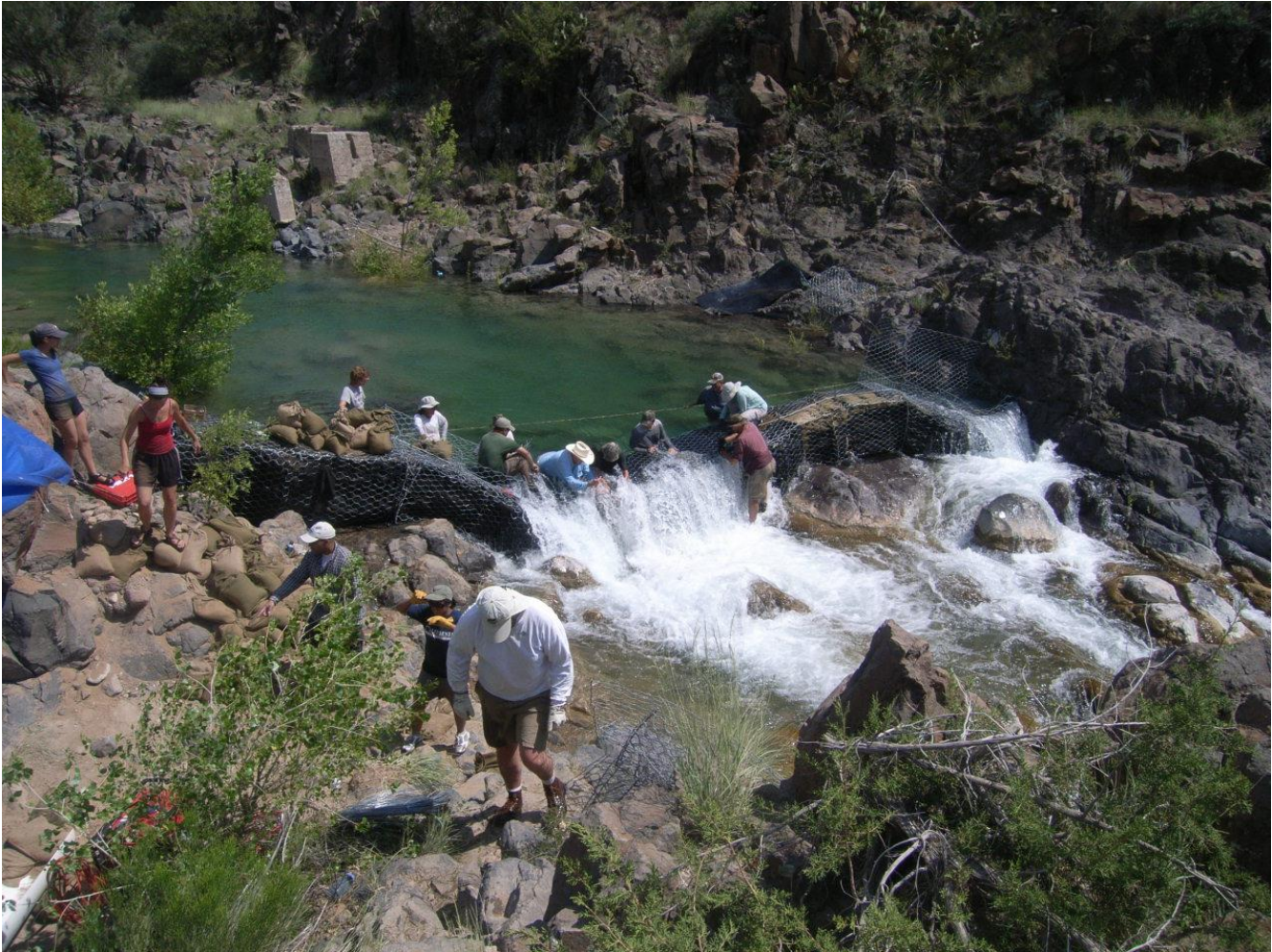
Figure 6. Construction of temporary fish barrier at Fossil Creek.
