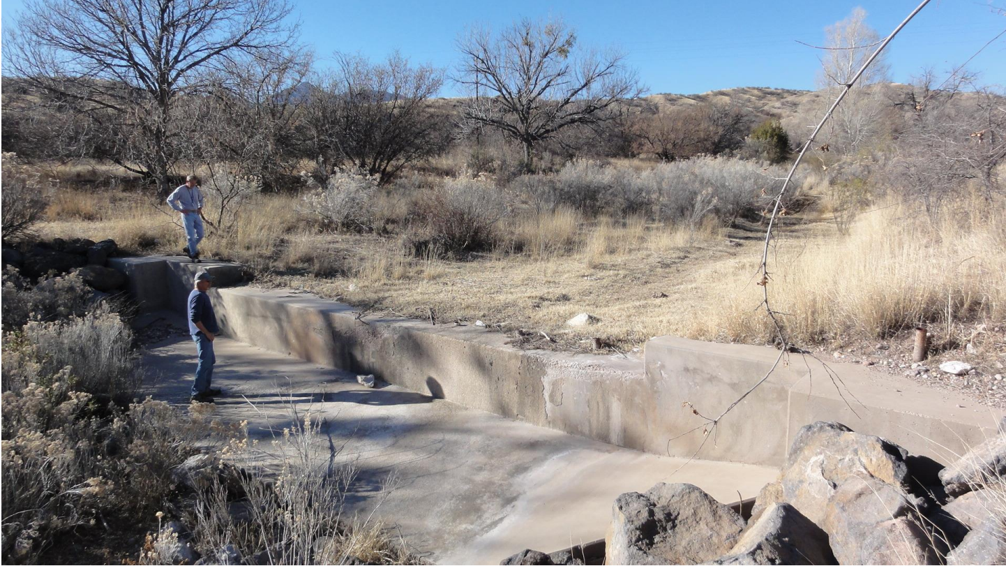
Figure 5. Cottonwood Springs Fish Barrier.
