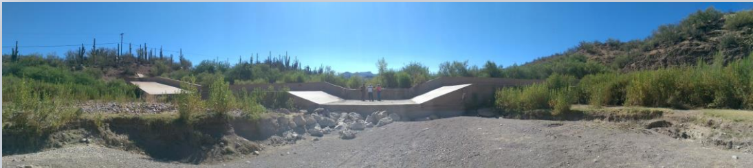
Aravaipa Creek Fish Barrier
