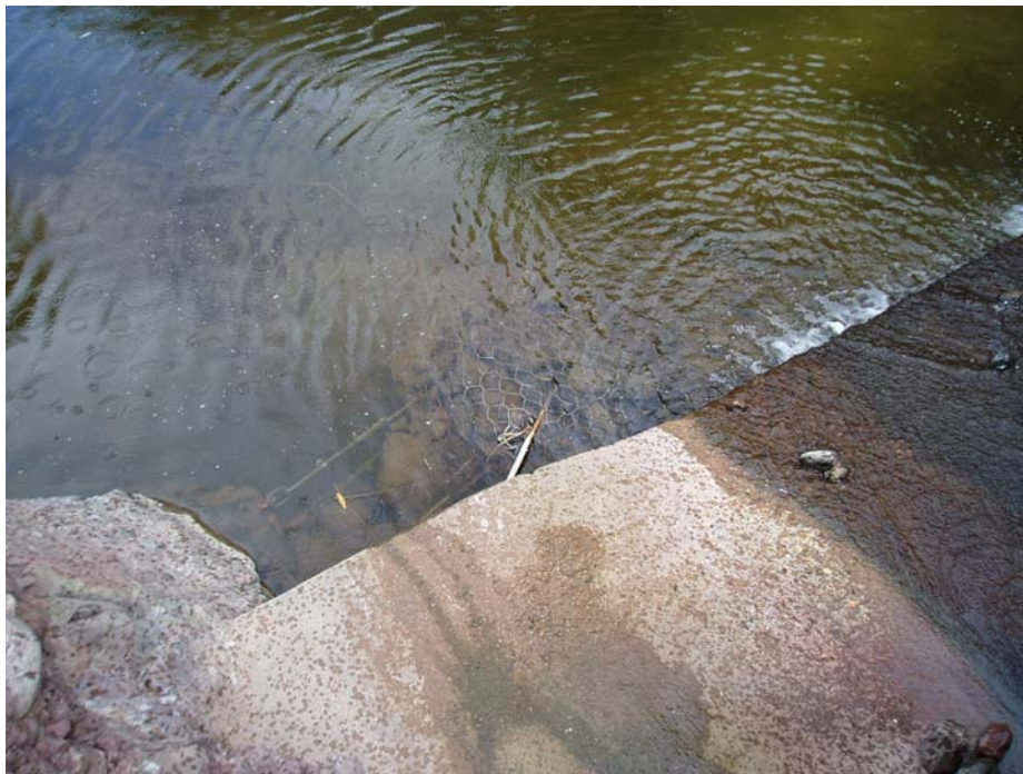
Fig. 4. Hot Springs Canyon, Cochise Co., Arizona, showing exposed wire gabion at the base of the constructed fish barrier apron on river left; October 11, 2012.
