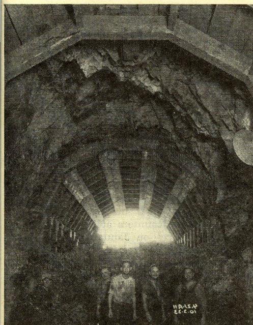
Picture at left shows "holing" through of first short section of tunnel in Coachella division of Aqueduct. Middle, east portal of Coxcomb tunnel showing picturesque "chimney rock." Right, east portal of Bernasconi tunnel, reached by heavy access cut.
