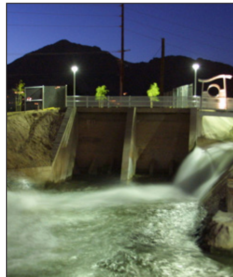
Waterworks at Arizona Falls, Phoenix, Arizona.
