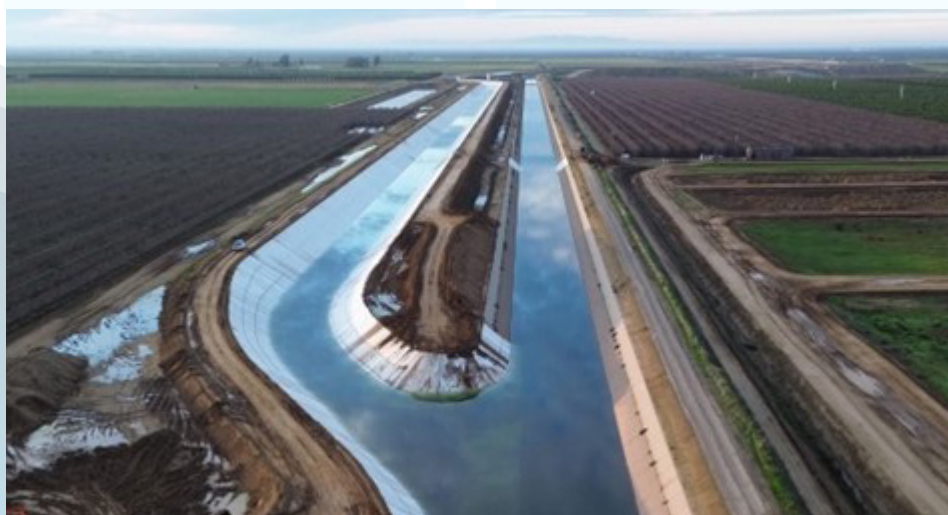
Newly constructed Friant-Kern Canal (left) and existing canal (right), Friant Division, Central Valley Project, California.
