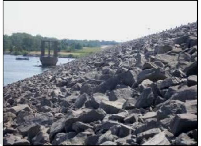
**Photo 2** – Fort Cobb uncontrolled glory-hole spillway. Releases when elevation is above flood pool.
