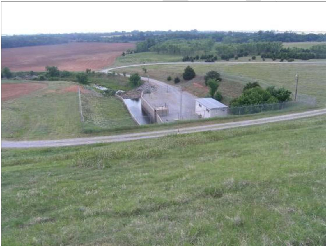
**Photo 3** – Downstream side of Fort Cobb Dam looking down on River Outlet Works chute and M&I sleeve-valve at start of pipeline delivery system.
