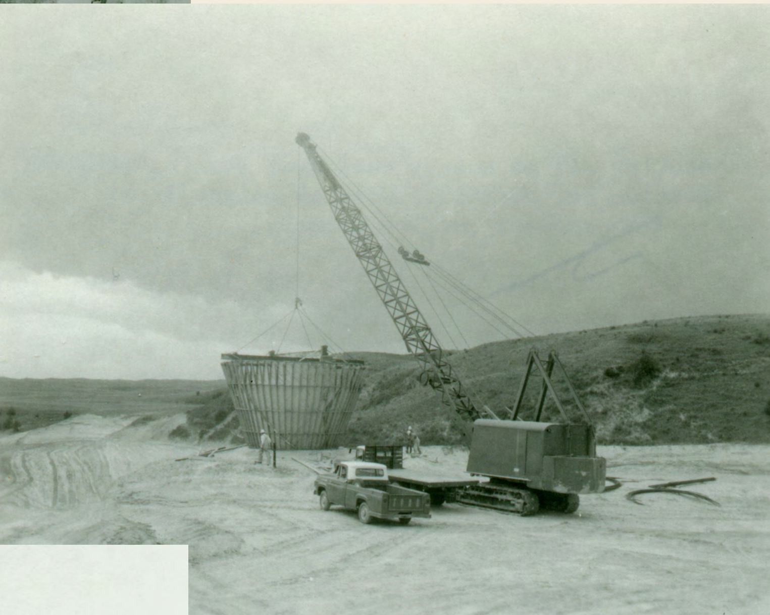
A dragline is setting the form in place for the morning glory section of the spillway inlet structure during June 1963.
