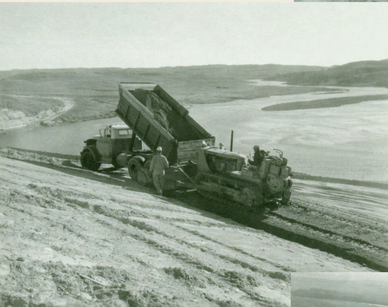
A Jersey spreader lays down soil cement facing on Merritt Dam in November 1963.
