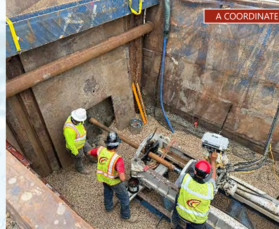
Crews preform a pilot bore for the City of Fort Pierre waterline, crossing Highway 14.
