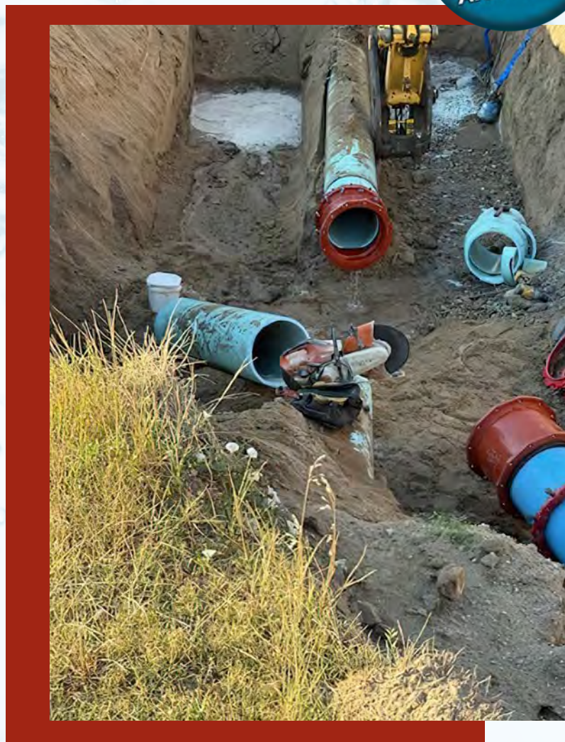
Crews work to feed a 12-inch pipe into the already placed 24-inch casing pipe that crosses Highway 14 for the City of Fort System.
