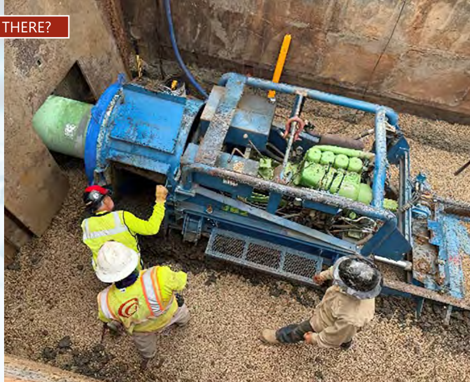
Crew places 24-inch steel casing pipe for 12-inch City of Fort Pierre waterline.
