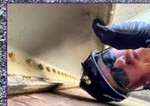
Carter Gulsvig inspects the bottom of the radial arm gate.
