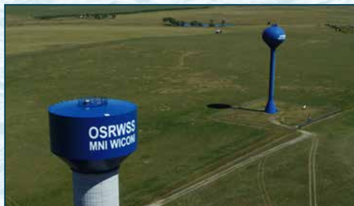
Aerial photograph of the OSRWSS Core System. The new 800,000 gallon tank in foreground and legacy tank in the background.
