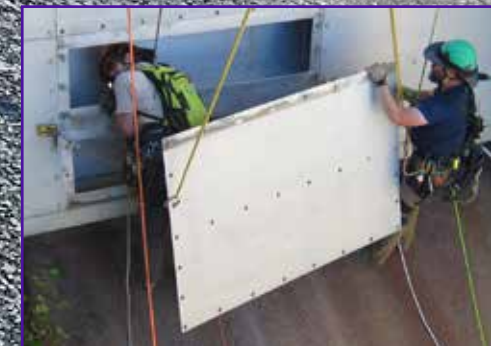
David Tordonato performs a radial gate interior inspection. Seth Joramo bracing the removed panel.
