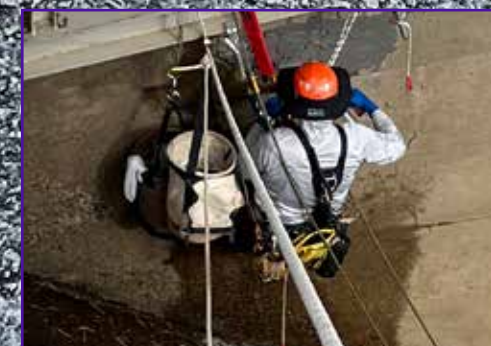
Adam Northrup repairs concrete at Olympus Dam.
