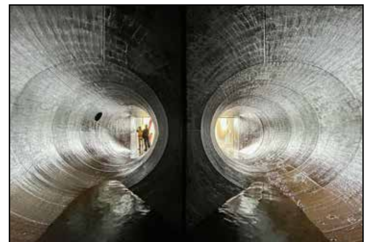
CR Team inspects the dewatered outlet works of Twin Lakes Dam, Colorado Photo by Adam Northrup
