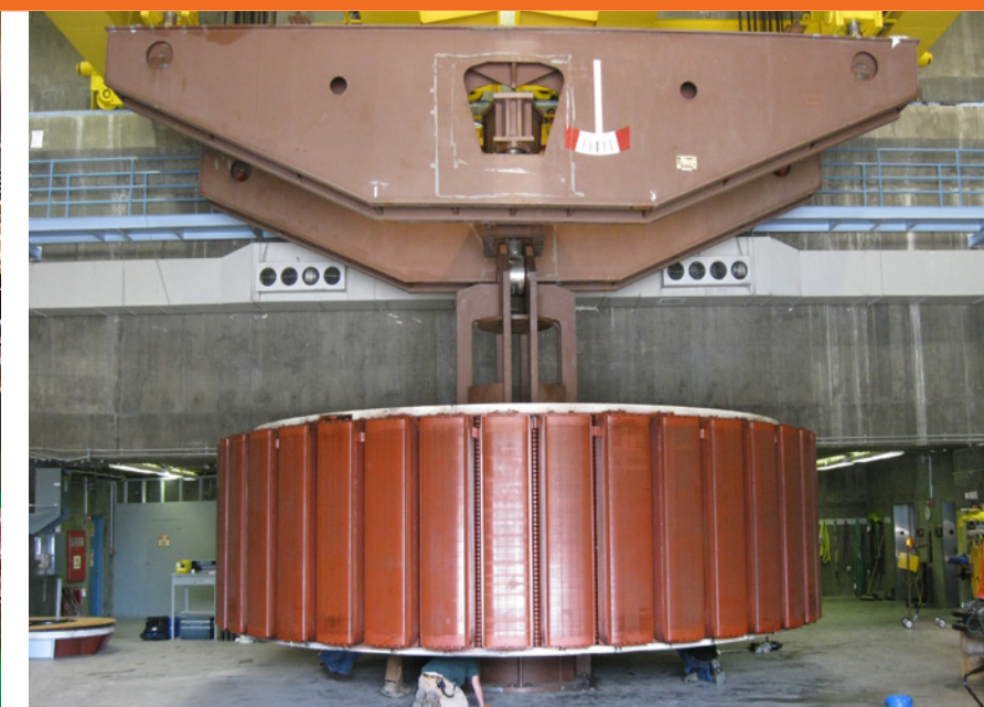
Rotor removed and on plant floor
