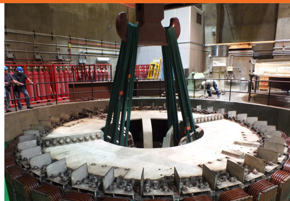
Rotor being removed from unit
