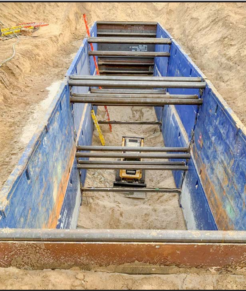
Trench box assembly in use at Fort Laramie Canal Tunnel No. 2, August 23, 2019. (G.T. Hastings)
