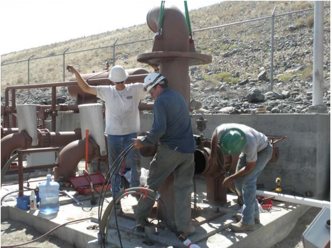
(Above) Workers guide electrical cables as the pump assembly is lowered into place at the Diamond Creek Pumping Plant, near Buffalo Bill Reservoir in northwestern Wyoming.
