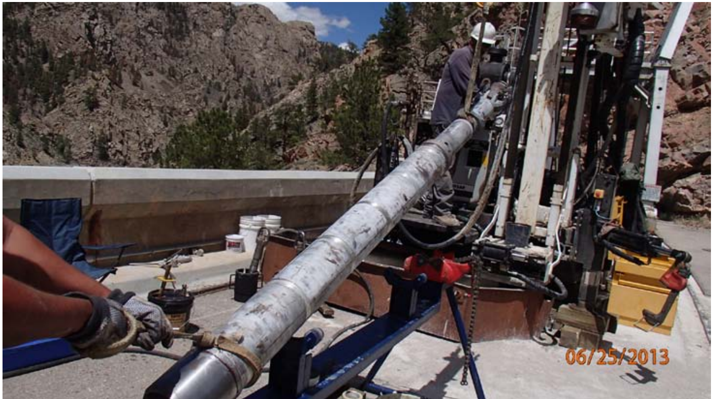
The exploration crew is preparing to hoist the double-tube core barrel assembly with cutting bit and lower it back into the bore hole.
