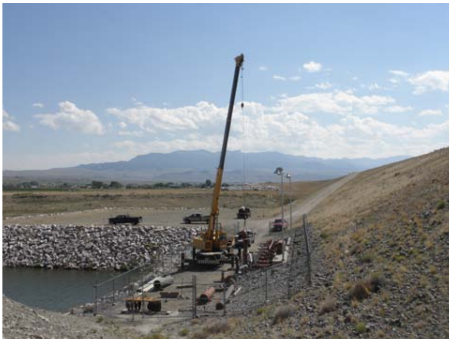
(Above) The crew lowers the pump assembly into the well (looking south along the east face of Diamond Creek Dike).
