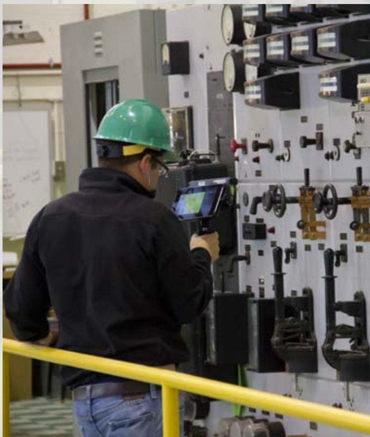
A member of the CyArk team uses a hand-held device to record detail of the original Shoshone Power Plant control panel. Digital images from multiple devices and angles will be combined to create an accurate 3D image map of both the interior and exterior of the plant.
