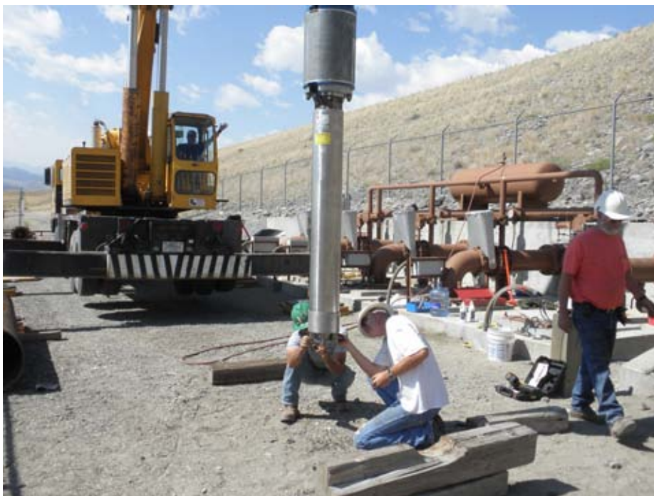
(Above) Crews inspect the pump assembly prior to installation.
