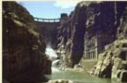
When completed on Wyoming's Shoshone River in 1916, Buffalo Bill Dam stood as an engineering marvel—one of the first concrete arch dams built in the United States. At 325 feet high, it also was the highest dam in the world at the time (surpassing New York's Croton Dam). Bureau of Reclamation
