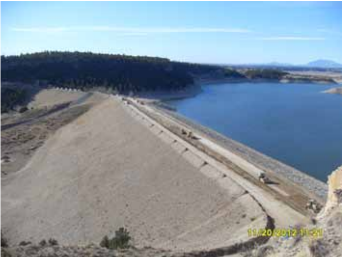
Placing embankment materials for the raising of Glendo Dam and construction of concrete parapet wall on the far side.
