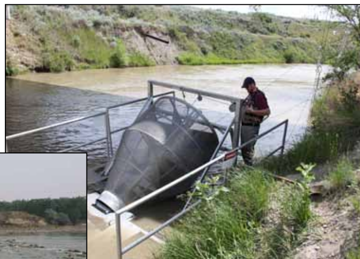
(Left) Intake Diversion Dam near Intake, Mont. (Above) Prior to canal screening, an average of 500,000 fish were annually entrained at Intake Diversion Dam.
