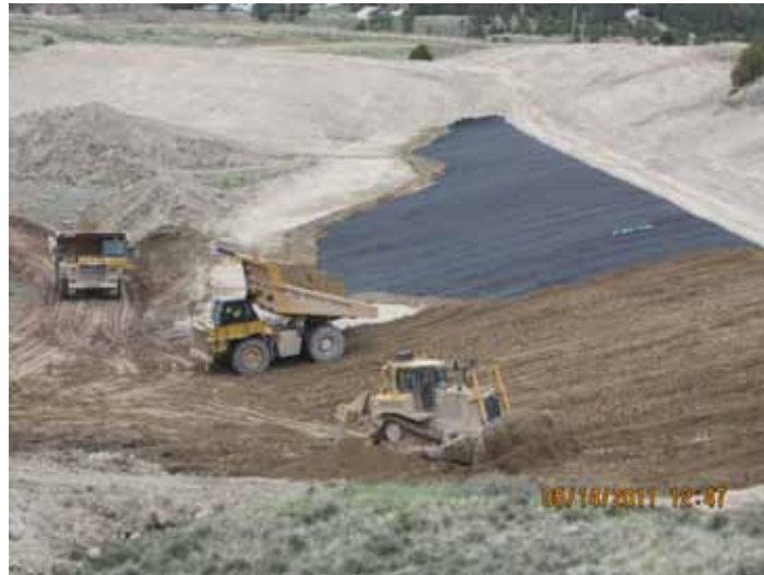
(Above) Workers placing miscellaneous fill material over geocomposite barrier on upstream slope of cofferdam.
