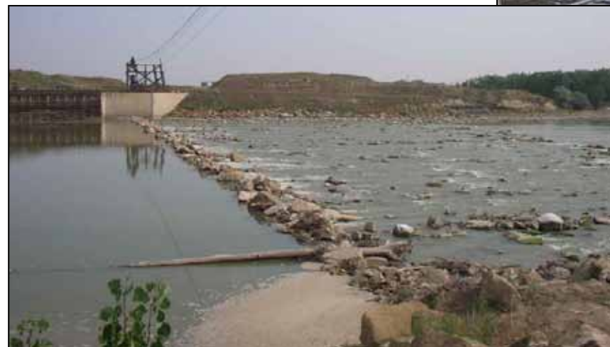
(Left) Intake Diversion Dam near Intake, Mont. (Above) Prior to canal screening, an average of 500,000 fish were annually entrained at Intake Diversion Dam.
