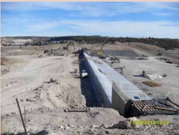
(Left) Placing roller-compacted concrete in the foundation trench for Glendo Dam’s auxiliary spillway. (Right) The crest section for the auxiliary spillway constructed on the roller compacted concrete.
