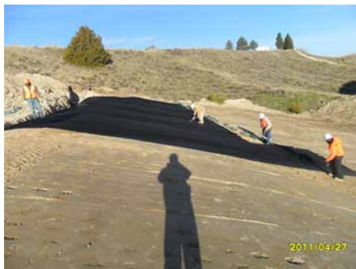
(Above) Workers installing geocomposite barrier on upstream slope of auxiliary spillway cofferdam.
