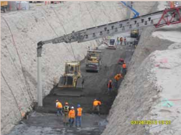
(Left) Placing roller-compacted concrete in the foundation trench for Glendo Dam’s auxiliary spillway. (Right) The crest section for the auxiliary spillway constructed on the roller compacted concrete.
