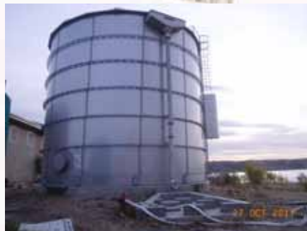
Construction of the 185,000 gallon Four Bears clear well.
