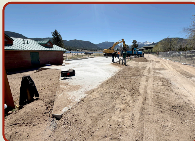
Decontamination station construction at Lake Estes. (Photo courtesy of Keith Williams, Estes Valley Recreation and Park District.)
