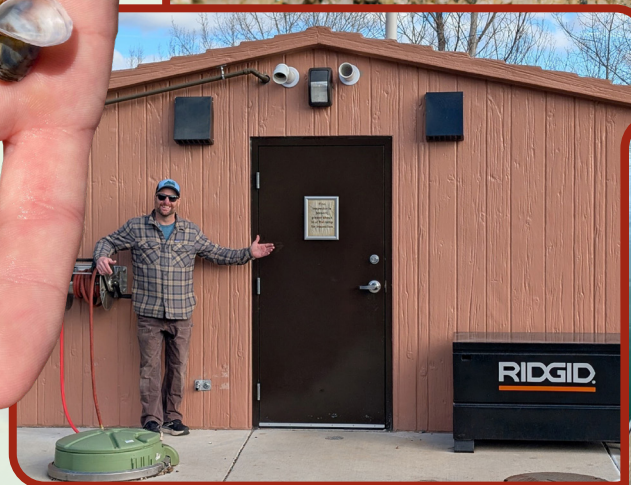
The South Bay wash pad station at Horsetooth Reservoir was completed this year. (Photo by Melissa Panella, ECAO.)
