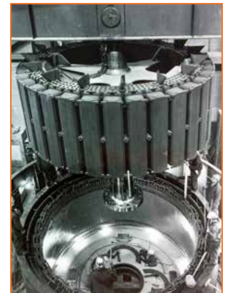
Rotor placement during original construction, Feb. 16, 1966, File photo by O. Gillen
