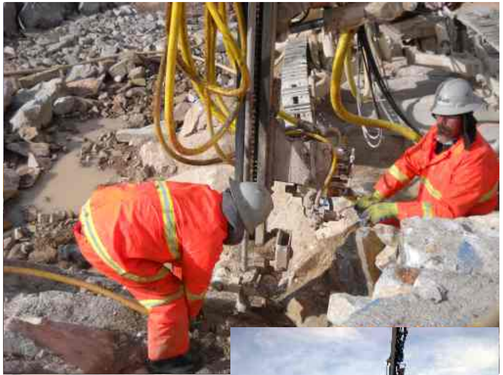
PREPARING FOR THUNDER: (Above) Crews drill holes for anchor bars to raise Pathfinder spillway. (Right) To increase reservoir storage, crews used heavy equipment and explosives to smooth and enlarge the natural granite spillway.
