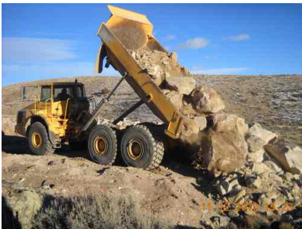
AFTER THE BLAST: (Above) Heavy equipment moves debris after crews blasted downstream from the extended spillway to widen the channel. Blasting work for the Pathfinder Dam modification consisted of fourteen different events between Nov. 17, 2010 and Jan. 11, 2011.
