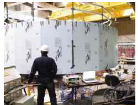
Workers insulate the rotor at Mount Elbert Powerplant in Colo. for heating in order to remove the spring keys.
