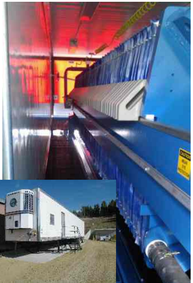
(Above) Reclamation's Leadville Water Treatment Plant uses this new sludge filter press to compact waste into "cakes" for transportation to a special environmental disposal site. The sludge filter press is self-contained in its own trailer on site (lower left).
