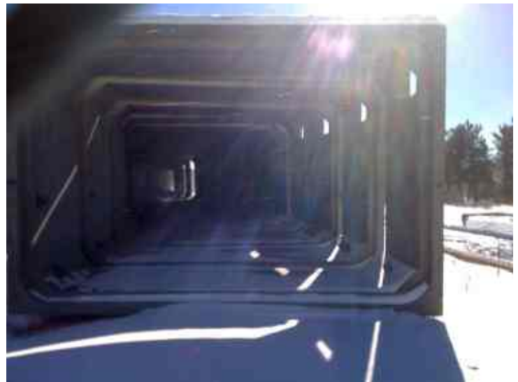
(Above) Delivered box culverts await installation alongside the open Pole Hill Canal.
