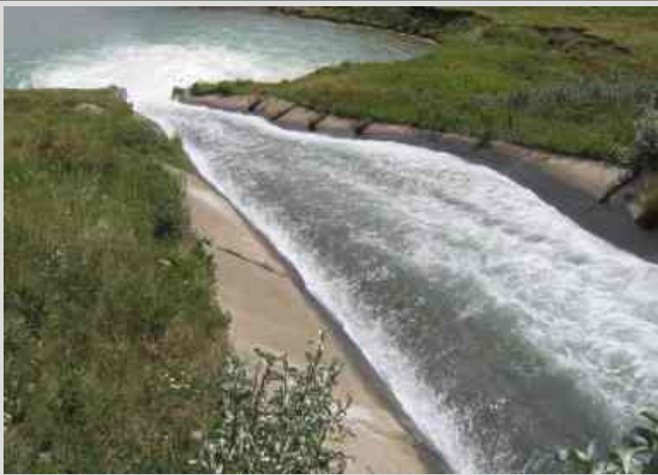
(Above, left) St. Mary Drop 4 Chute on the Milk River Project, east of Glacier National Park, Mont., drops 66 feet in elevation. It is one of a series of five major drops within a distance of two miles. (Above, right) Woodston Diversion Dam weir, in north central Kansas, drops 13 feet in elevation depending on upstream and downstream water surface elevations.
