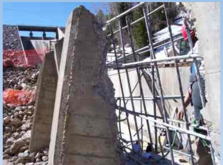
(Left) Work on the spillway at Green Mountain Dam included painting the spillway gates. (Above) Concrete replacement on the Green Mountain spillway included rebuilding whole sections of spillway walls. (Right) Moltz Construction also patched voids up and down the spillway.
