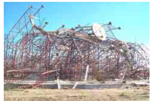
BEFORE AND AFTER: The partially completed main water treatment plant tower on the Lewis and Clark Rural Water Project in South Dakota, before and after a “microburst” storm pounded the area with hail and high winds.
