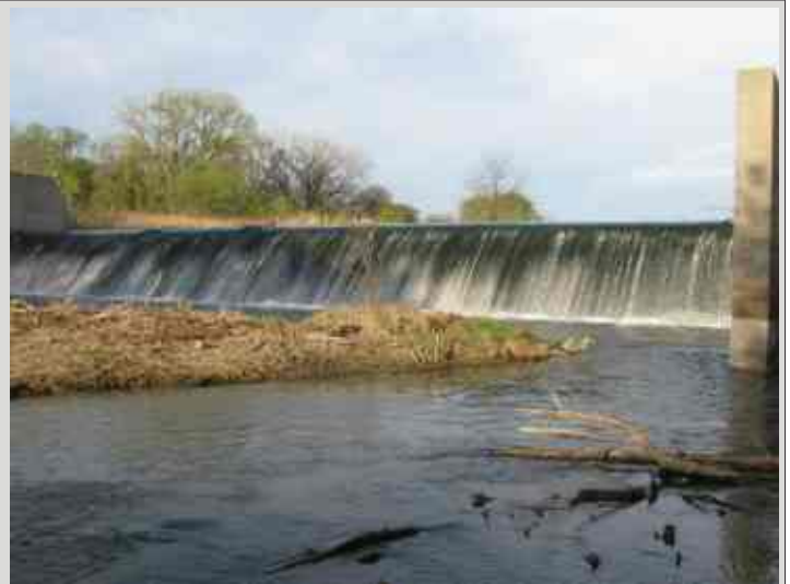
(Above, left) St. Mary Drop 4 Chute on the Milk River Project, east of Glacier National Park, Mont., drops 66 feet in elevation. It is one of a series of five major drops within a distance of two miles. (Above, right) Woodston Diversion Dam weir, in north central Kansas, drops 13 feet in elevation depending on upstream and downstream water surface elevations.
