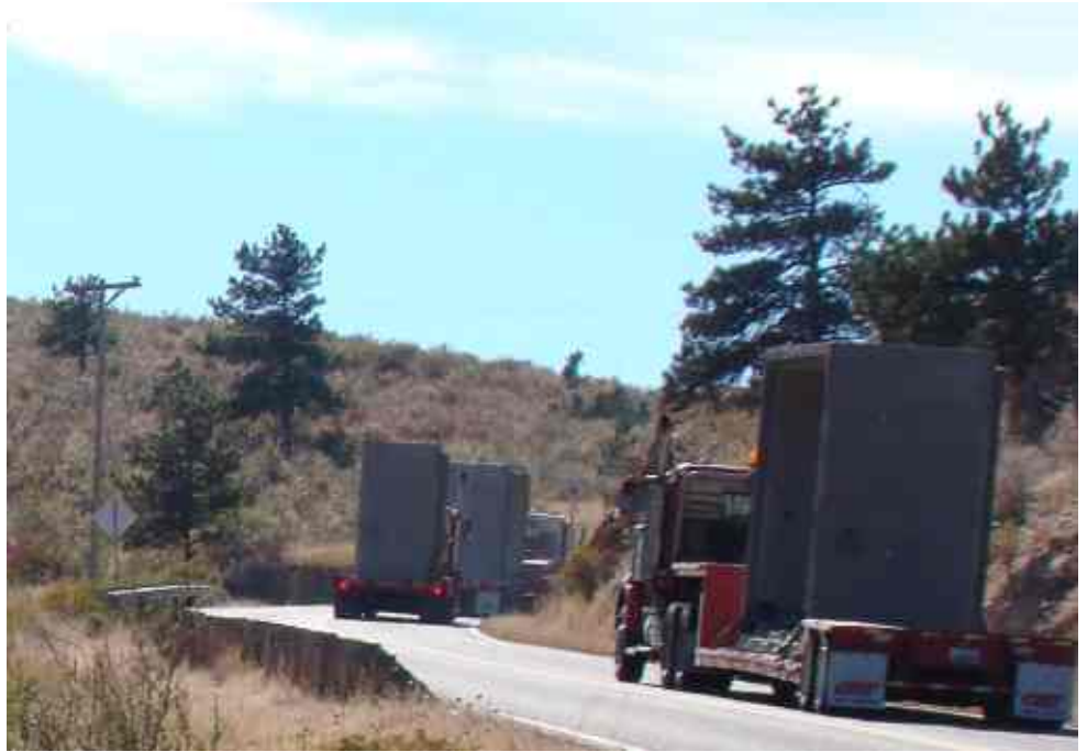
(Above) Hauling of the Pole Hill box culverts was done in multiple delivery trips of four trucks at a time, with each flatbed truck carrying a single, 20 ton box culvert.
