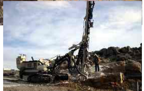
PREPARING FOR THUNDER: (Above) Crews drill holes for anchor bars to raise Pathfinder spillway. (Right) To increase reservoir storage, crews used heavy equipment and explosives to smooth and enlarge the natural granite spillway.
