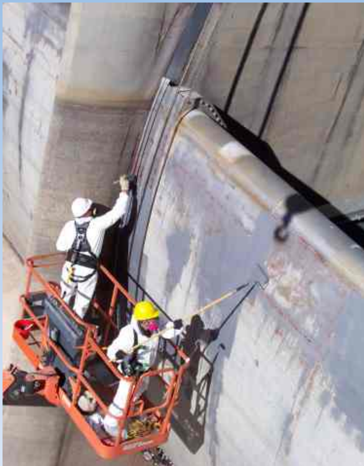
(Left) Work on the spillway at Green Mountain Dam included painting the spillway gates. (Above) Concrete replacement on the Green Mountain spillway included rebuilding whole sections of spillway walls. (Right) Moltz Construction also patched voids up and down the spillway.
