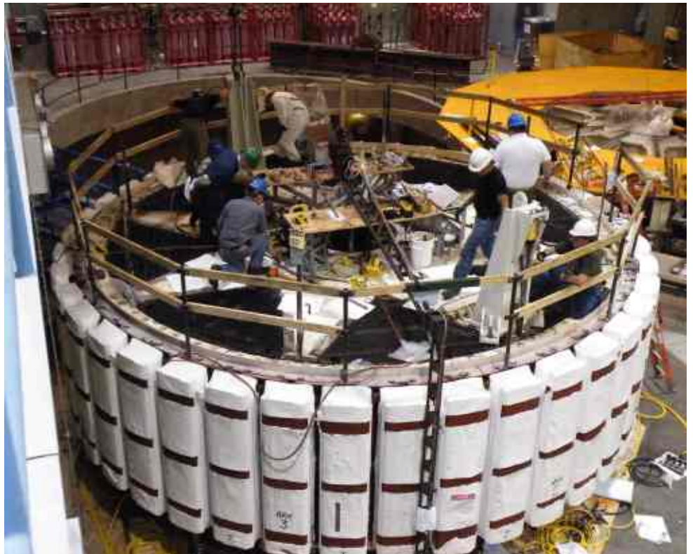
Workers insert keys with strongbacks using hydraulic rams at Mount Elbert Powerplant, Colo.
