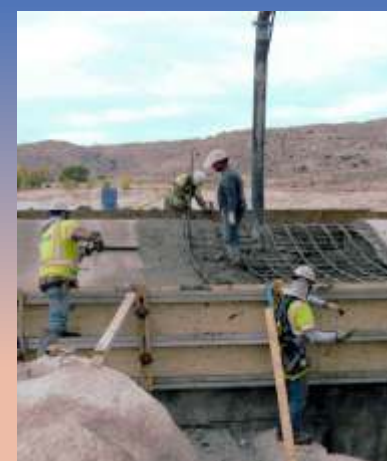
Finishing the new concrete spillway crest at Pathfinder Dam.
