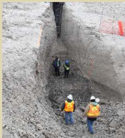
Engineers inspect excavation of the embankment at Red Willow Dam in Nebraska as repairs begin under the Safety of Dams Program.
