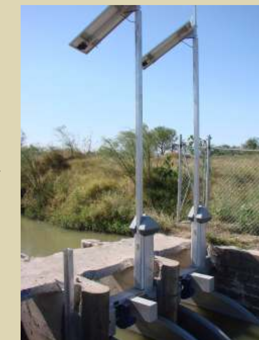
WaterSMART funded Rubicon gate and telemetry system for Cameron County Irrigation District No. 2 on the Rio Grande in southern Texas.
