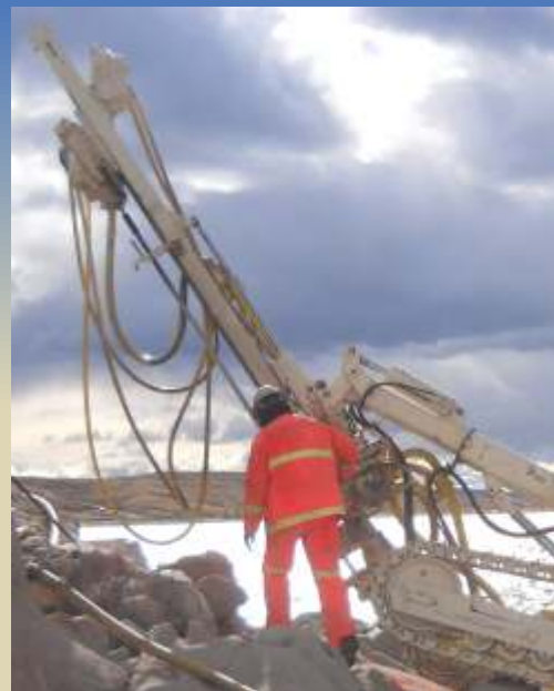
Preparation for blasting for Pathfinder Dam's spillway modification. Pathfinder Reservoir now can store more water to meet the needs of Wyoming and to provide habitat along the Platte River in Nebraska.
