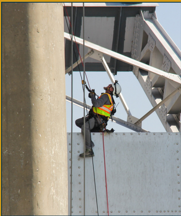
Joel Finch, MB Region civil engineer, inspects a Webster Dam spillway radial gate in Kansas. Photo by Mike Rauh
