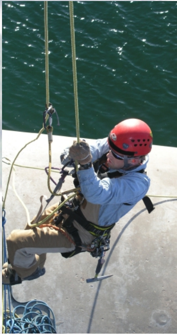
Engineers with special training use climbing gear to inspect dams and other facilities.
