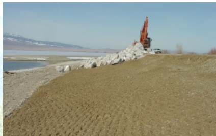
Protective lining and rock covering is added to the dikes at Canyon Ferry.
