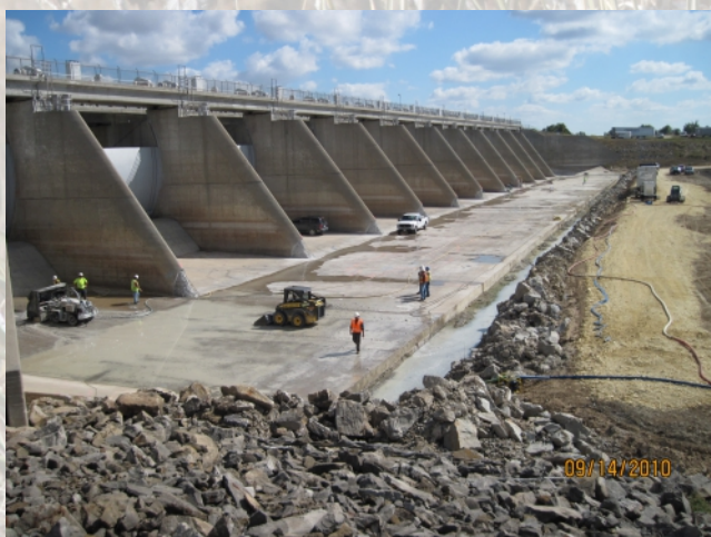
Spillway structure concrete repairs at Glen Elder Dam in Kansas were the first in the region to use hydrodemolition (the use of high pressure water) for removal of deteriorated concrete.
