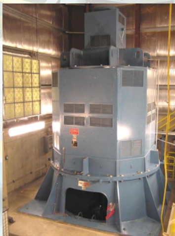
(Left) Tiber LLC's 7.5 Mw generator installed at Tiber Dam in Montana.
