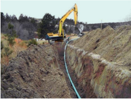
Installation of water line on the Mni Wiconi Rural Water System in South Dakota.
