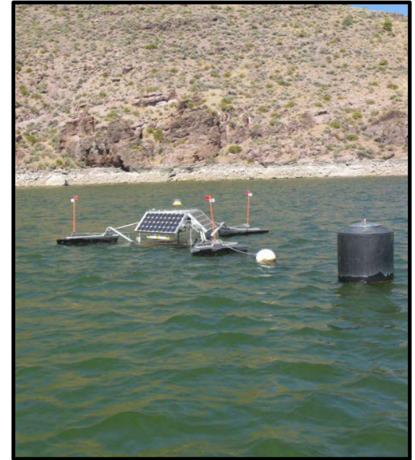
Solar pump operating at Newcastle Reservoir, Utah
