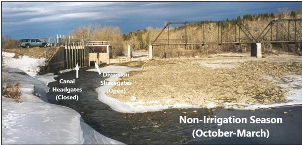
**Figure 3.** St. Mary Diversion Dam during the non-irrigation season. Photo taken from St. Mary River upstream of diversion dam and headworks (BOR 2020).
