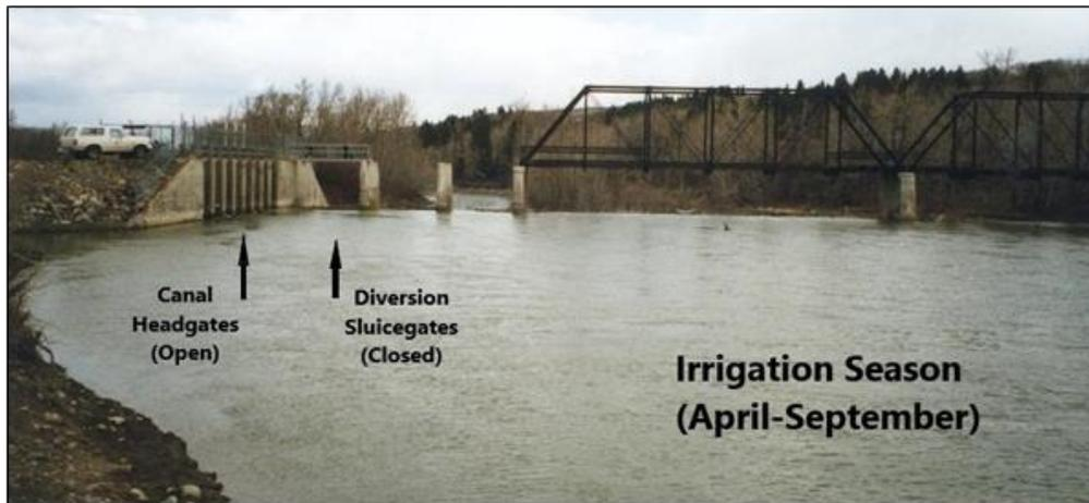
**Figure 4.** St. Mary Diversion Dam during the irrigation season. Photo taken from St. Mary River upstream of diversion dam and headworks (BOR 2020).
