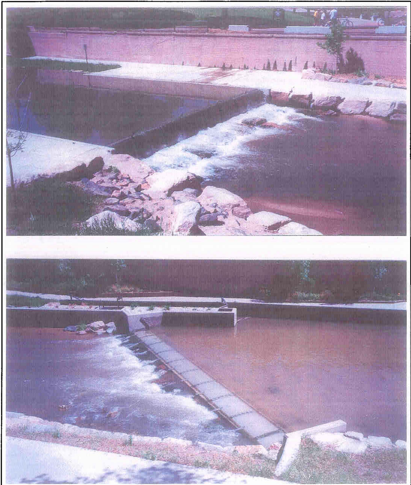
Figure 8. Obermeyer Weir Photos
