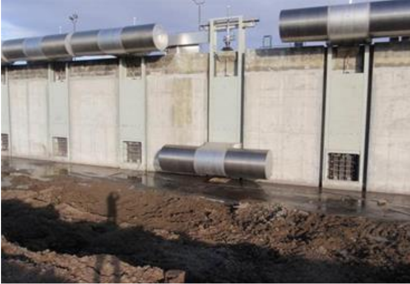
Figure 3. New Intake Headworks structure under construction showing the river side with Intake Screens, Inc. fish screens (ISI T78-100 Tee Screen) over intake inlet conduit while the others are in the up position (photo from Intake Screens, Inc.).
