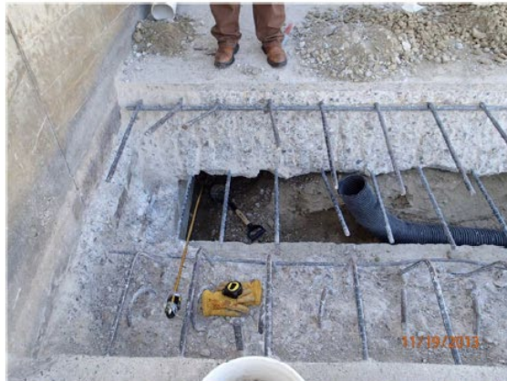
2013 Spillway slab repair at station 10+63.50 (left). Void found near right wall looking upstream from station 10+63.50 (below).
