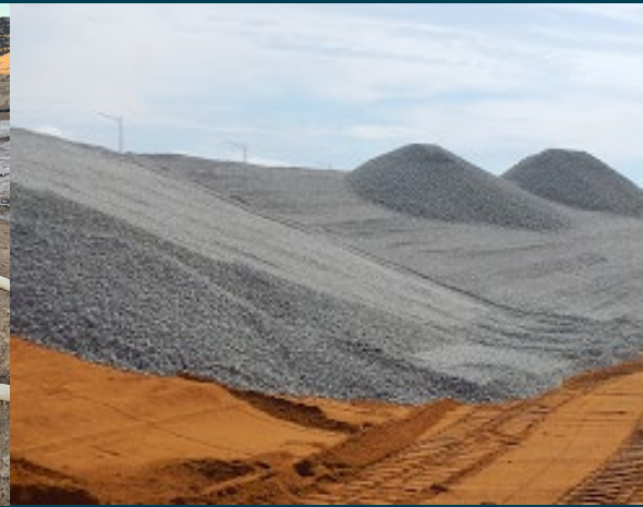
Step 2: Install Sand Filter and Gravel Drain
