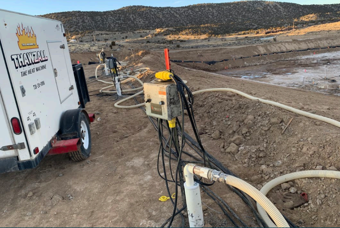
Step 1: Install Dewatering and Excavate Sand Filter Trench
