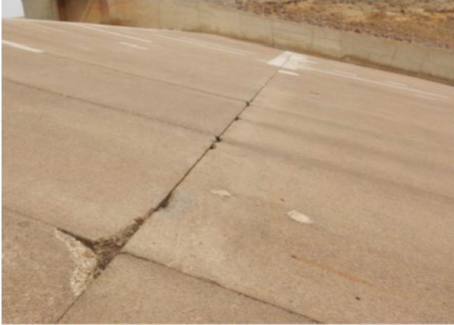
Figure 25.—Concrete damage creating unfavorable transverse offset for spillway flows (facing left) (CR photo CE-45) [2]
