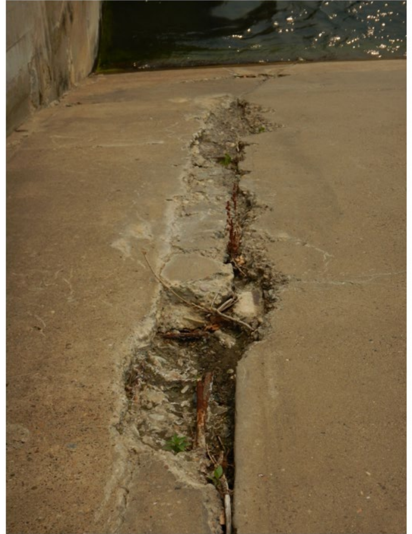
Photo CE-43 – Fresno Dam – Severe concrete damage and exposed steel rebar on left side of spillway chute slab (near stilling basin, facing downstream). 8/15/2018
