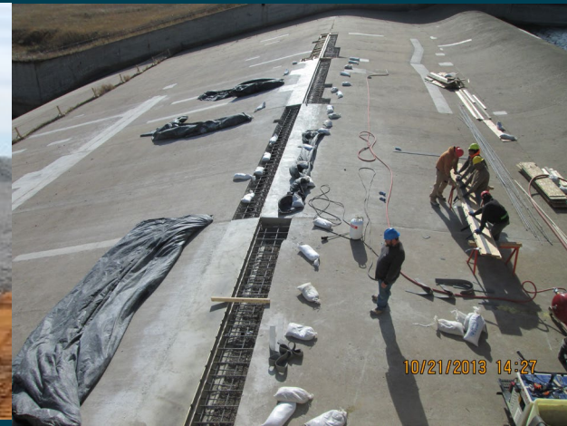
Step 3: Replace Spillway Joints
