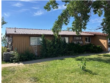
Concession Building - Exterior
