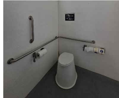
Vault Toilet - Interior
