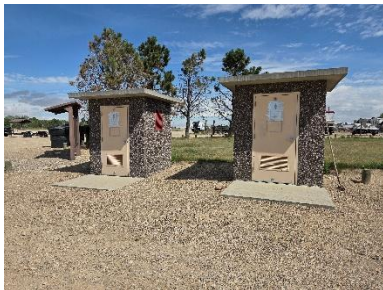
Vault Toilet - Exterior
