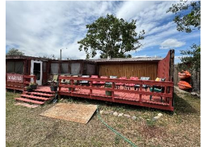
Concession Building - Exterior
