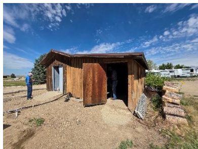
Utility Building - Exterior
