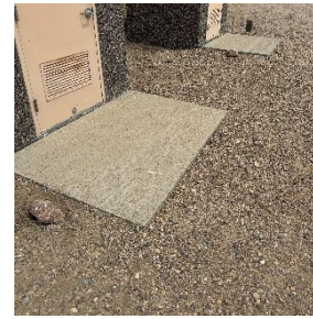
Vault Toilet - Exterior
