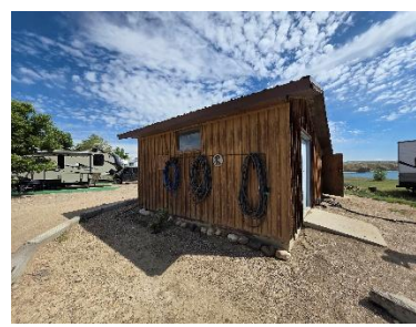
Utility Building - Exterior
