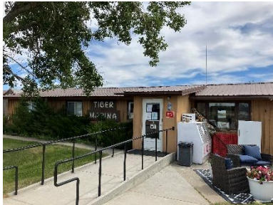
Concession Building - Exterior
