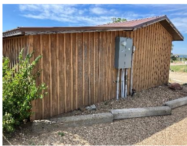
Utility Building - Exterior
