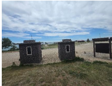
Vault Toilet - Exterior
