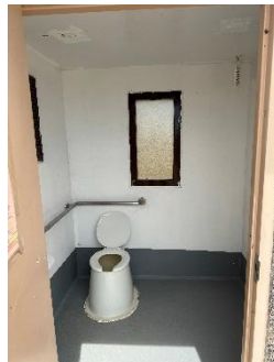
Vault Toilet - Interior
