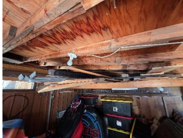
Utility Building - Interior
