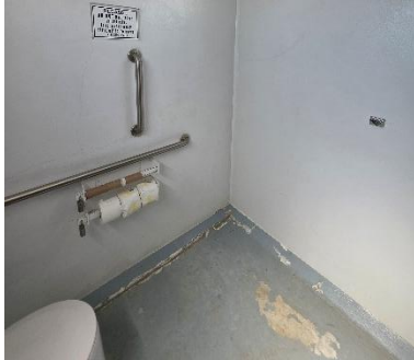
Vault Toilet - Interior
