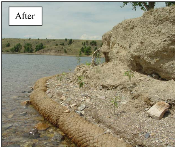
Figure 3. Cave Point is a site where Reclamation has implemented and is monitoring shoreline stabilization measures, including a coir log and cottonwood/willow plantings.
