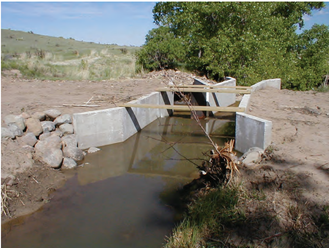
Figure 3. Splitter box located at measurement site SS07 on the Enlarged Southside Canal.
