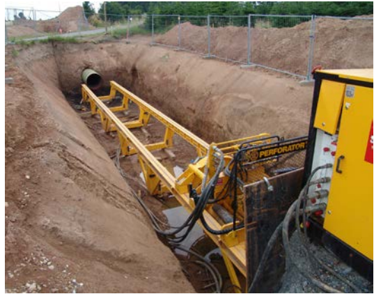
Photo 2-11. Trenchless construction techniques could be used to avoid disturbing major roadways, streams, and other resources
