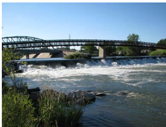
Photo 2–8. The River South Alternative river intake location would be near the Arkansas River at Moffat St. gage. A new diversion structure may be needed.
