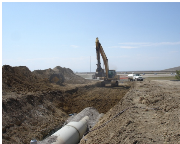
Photo 1–3. The AVC would be a buried pipeline, similar to the one shown in this photo, and would convey water from Pueblo Reservoir east to Lamar
