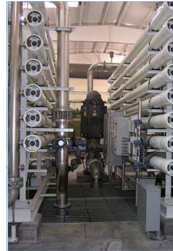
Photo 2-2. Tubular modules and pump at La Junta's existing reverse osmosis water treatment facility
