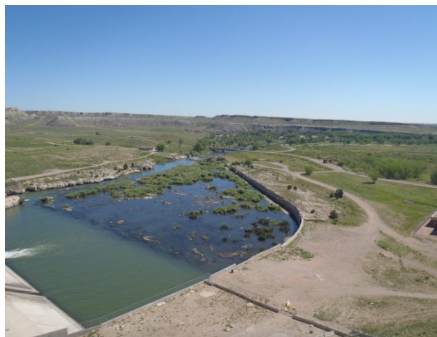
Photo 1–4. The Interconnect pipeline would connect the existing Pueblo Reservoir south outlet works manifold (bottom-right of photo, below ground) to the north outlet works
