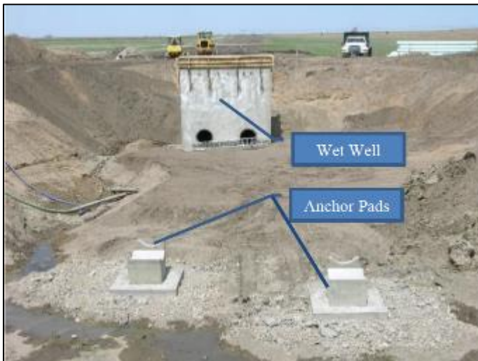
Figure 6. Example of Wet Well and Anchor Pads.
