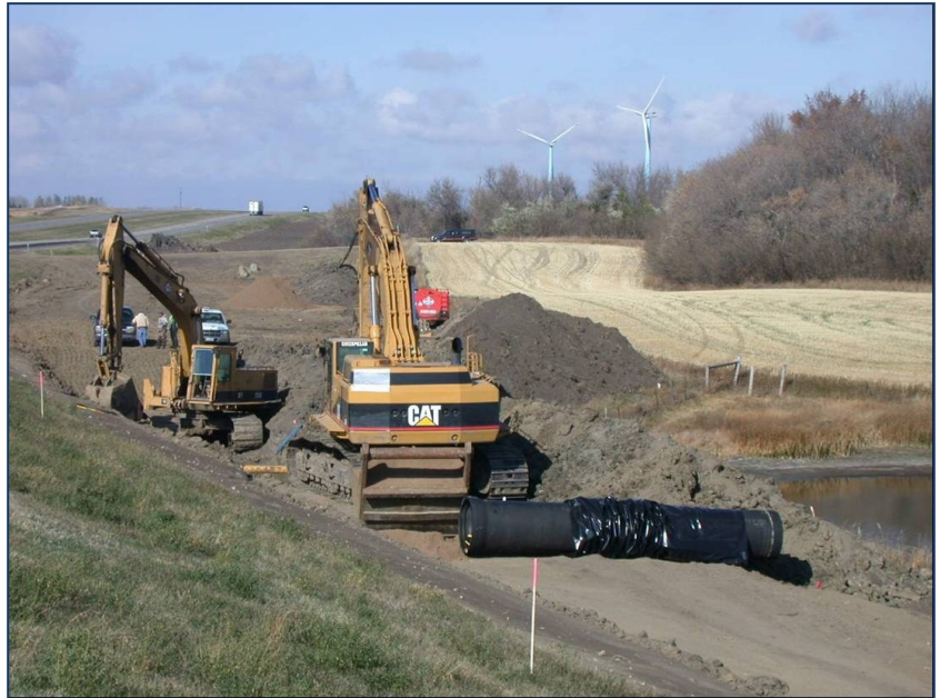
Construction of Project Main Transmission Pipeline
