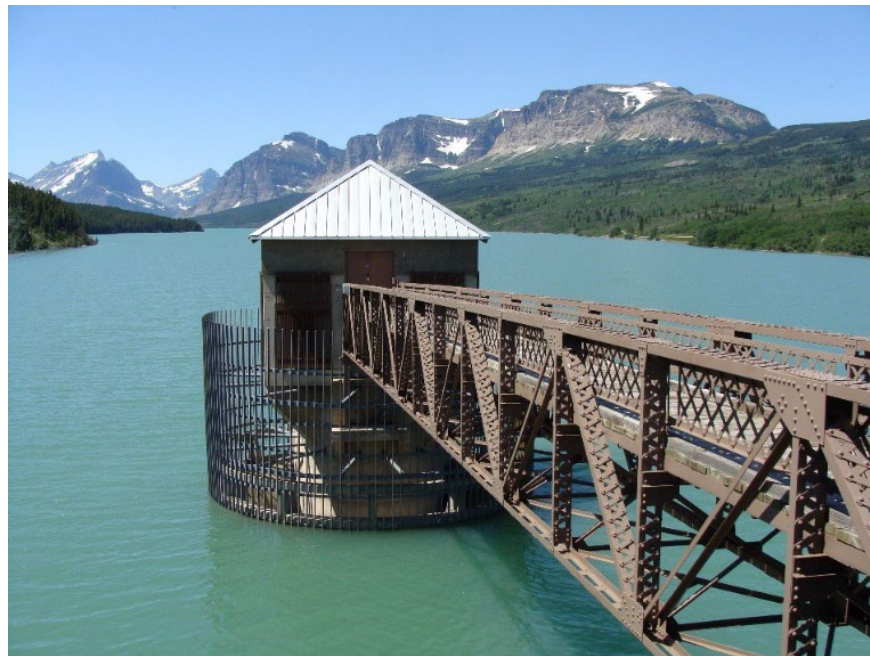
Figure MTG-28.—Lake Sherburne's outlet works.
