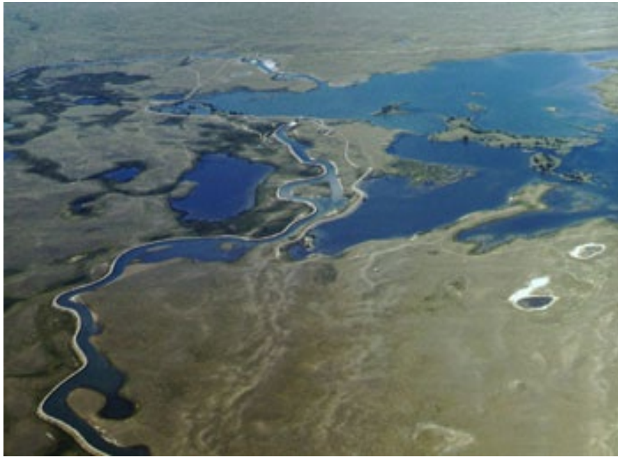
Figure MTG-15.—Aerial view of Pishkun Reservoir.
