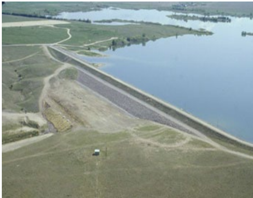
Figure MTG-13.—View of Helena Valley Reservoir and Dam.
