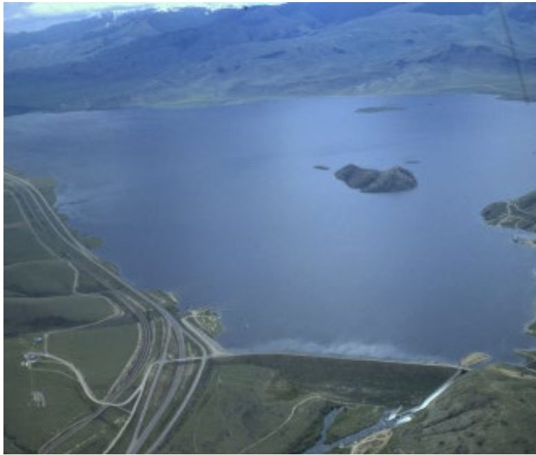
Figure MTG-2.—Aerial view of Clark Canyon Reservoir.
