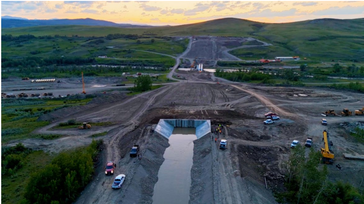
Figure MTG-29.—Completed St. Mary Canal Siphons.
