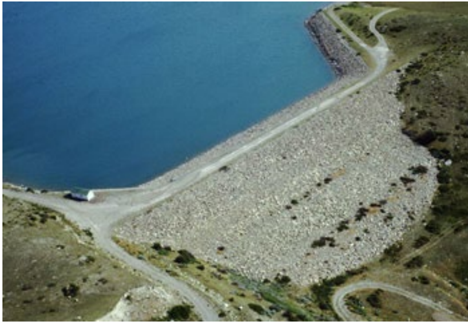
Figure MTG-16.—View of Willow Creek Dam and reservoir.
