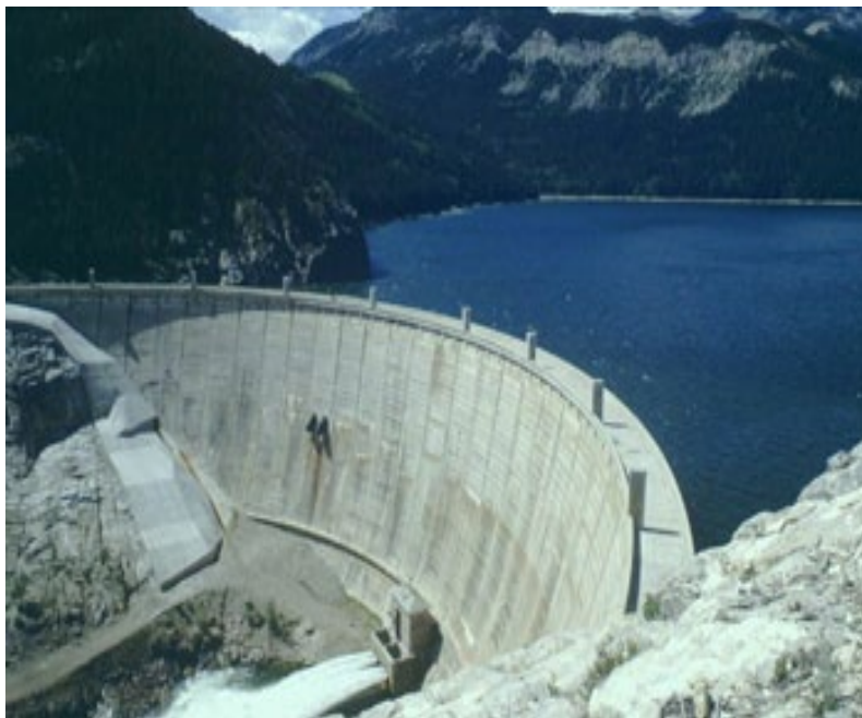
Figure MTG-14.—Gibson Reservoir and Dam.
