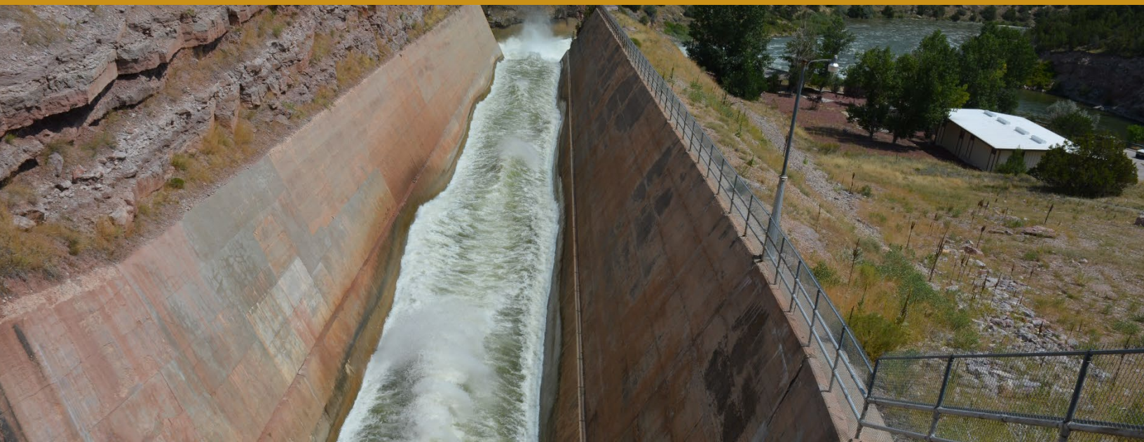
Guernsey Reservoir Spillway, Wyoming
