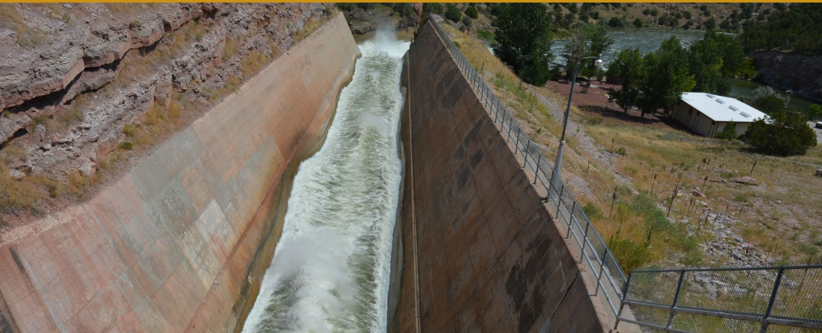
Guernsey Reservoir Spillway, Wyoming
