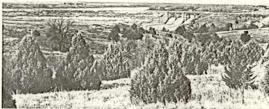
View of the downstream face of Medicine Creek Dam. Note the trees and grass over the general area. It takes as long as twenty years from the time of construction for grasses and trees to cover the scars of construction. The dam was placed in operation in 1949.
