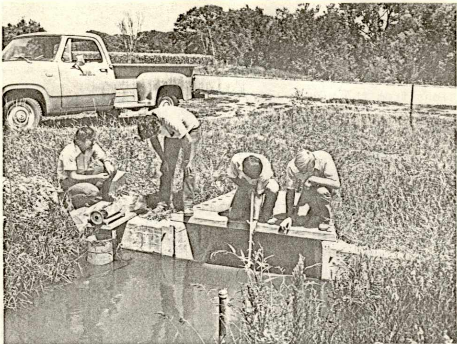
Special studies are being made on the Farwell Canal system operation to evaluate the efficiency. This water stage recorder was installed on an operational wasteway near Dannebrog, Nebraska.
