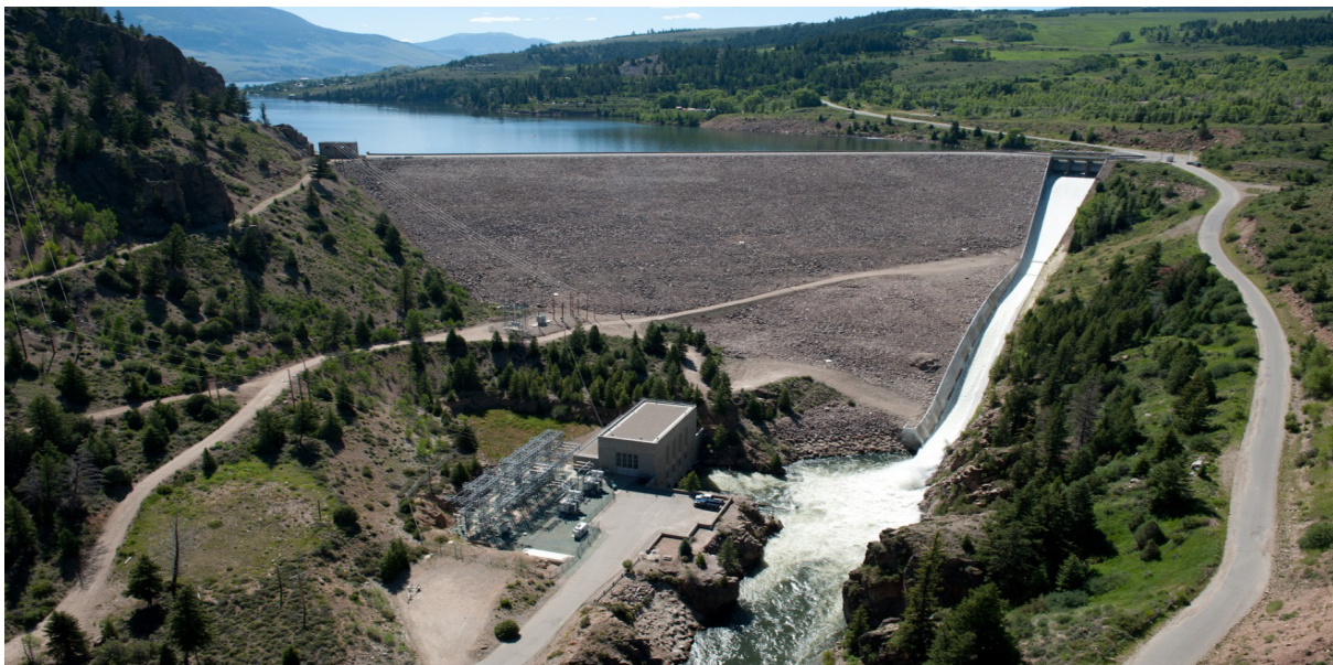
Photograph 1.—A summer release through the spillway at Green Mountain Dam and Reservoir. Green Mountain Powerplant, located just below the dam, is also generating power.
