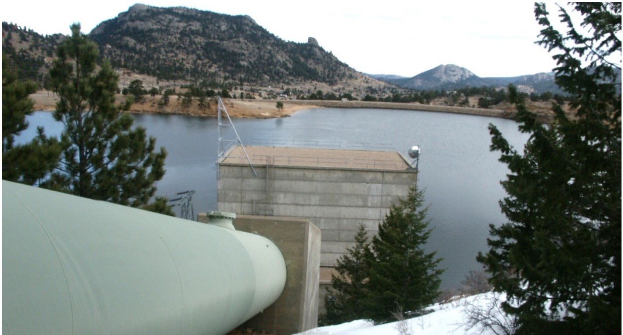
Marys Lake Penstock (left), Powerplant (center) and Marys Lake (background).
