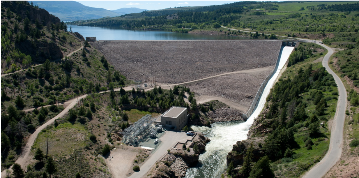
A summer release through the spillway at Green Mountain Dam and Reservoir. Green Mountain Powerplant, located just below the dam, is also generating power.
