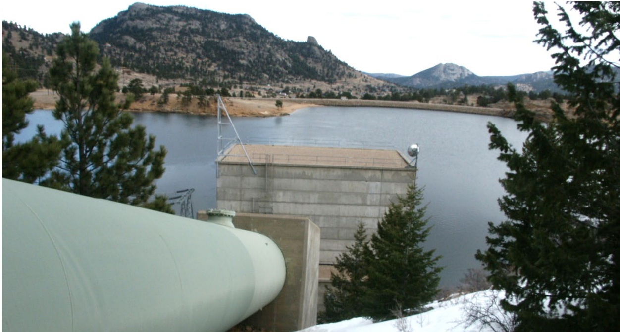
Figure 2: Marys Lake Penstock (left), Powerplant (center) and Marys Lake (background).
