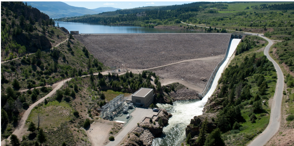
Figure 1: A summer release through the spillway at Green Mountain Dam and Reservoir. Green Mountain Powerplant, located just below the dam, is also generating power.
