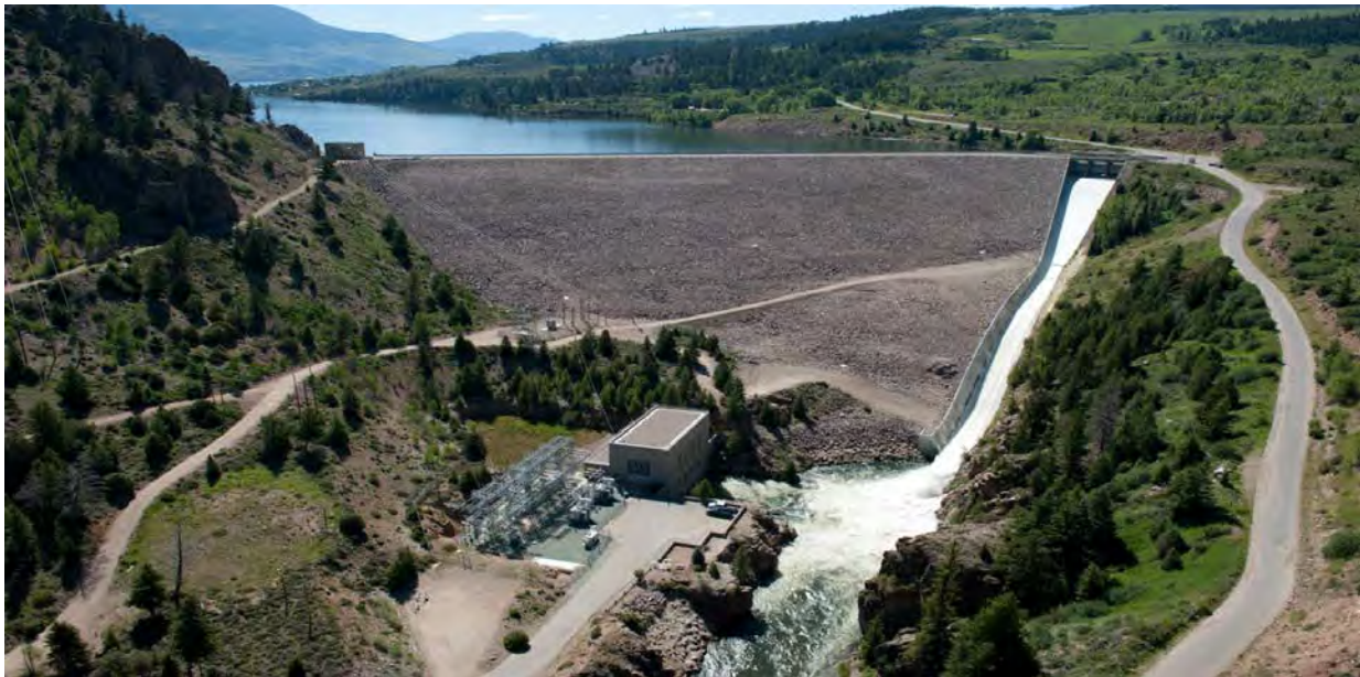
A summer release through the spillway at Green Mountain Dam and Reservoir. Green Mountain Powerplant, located just below the dam, is also generating power.
