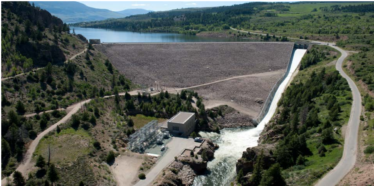
A summer release through the spillway at Green Mountain Dam and Reservoir. Green Mountain Powerplant, located just below the dam, also generating power.
