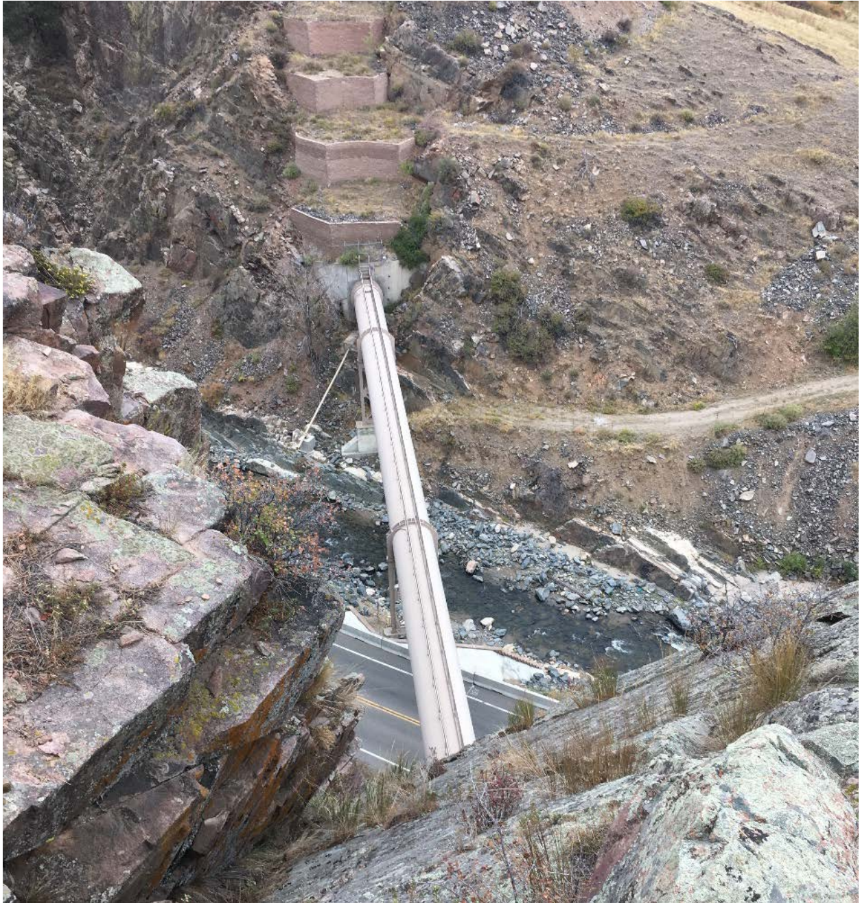
Big Thompson Siphon Connecting Charles Hansen Feeder Canal 930 and 550 Sections.
