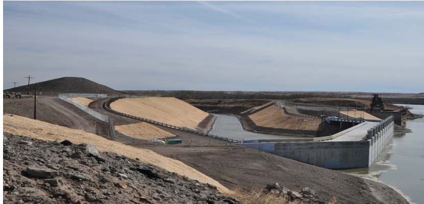
Figure 6: Lower Yellowstone Headworks and Fish Screen Structure (screens submerged)
