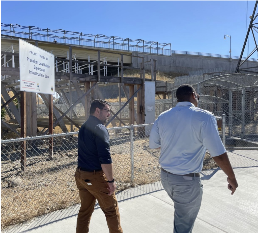
Nimbus Dam Fish Ladder nursery modernization, Central Valley Project, California. BIL-funded Extraordinary Maintenance of $10 million in FY 2023.
