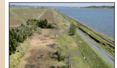
Figure 2: Photograph of Major Slumping of Landside Slope of Naruse River Right Levee and Approach Road at River Kilometer 30.0 (NSR 5307, E 141.0064, April 20, 2011) – see Figure 8 for additional views and aerial image
