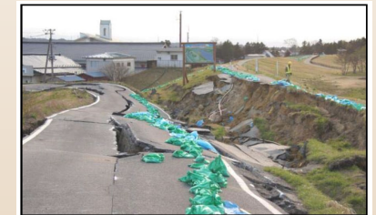
Figure 2: Photograph of Major Slumping of Landside Slope of Naruse River Right Levee and Approach Road at River Kilometer 30.0 (NSR 5307, E 141.0064, April 20, 2011) – see Figure 8 for additional views and aerial image
