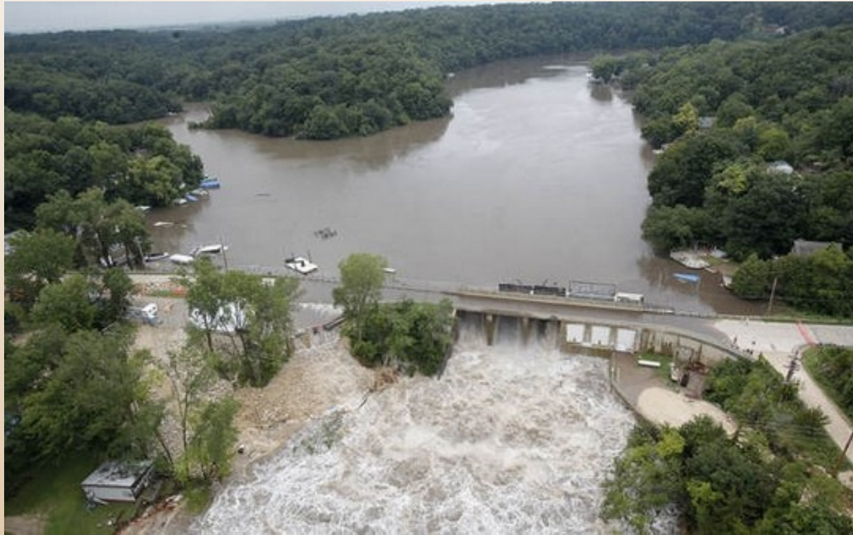
Lake Delhi Dam, Eastern Iowa July 24, 2010 Overtopping and Internal Erosion Failure (43 foot high embankment, 3,790 acre-ft)
