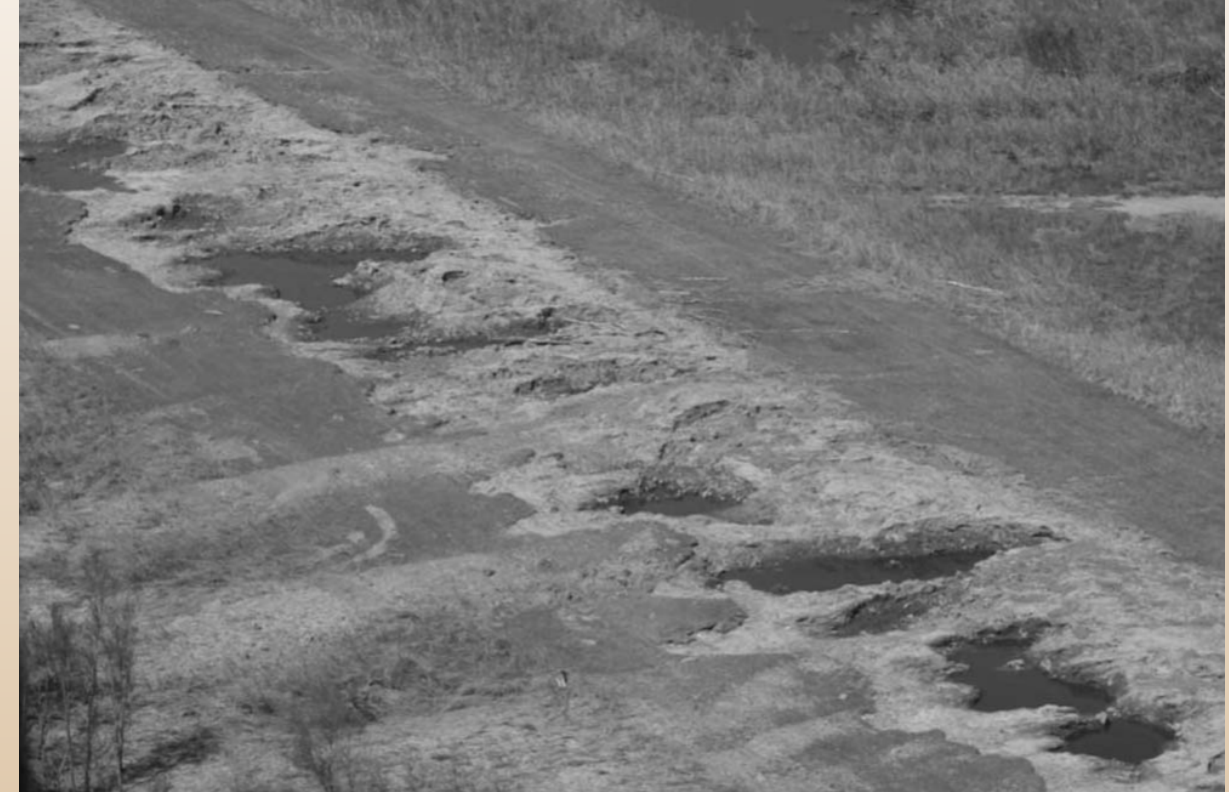
Catastrophically eroded levee section along the northeast frontage of the St Bernard Parish levee, MRGO channel
