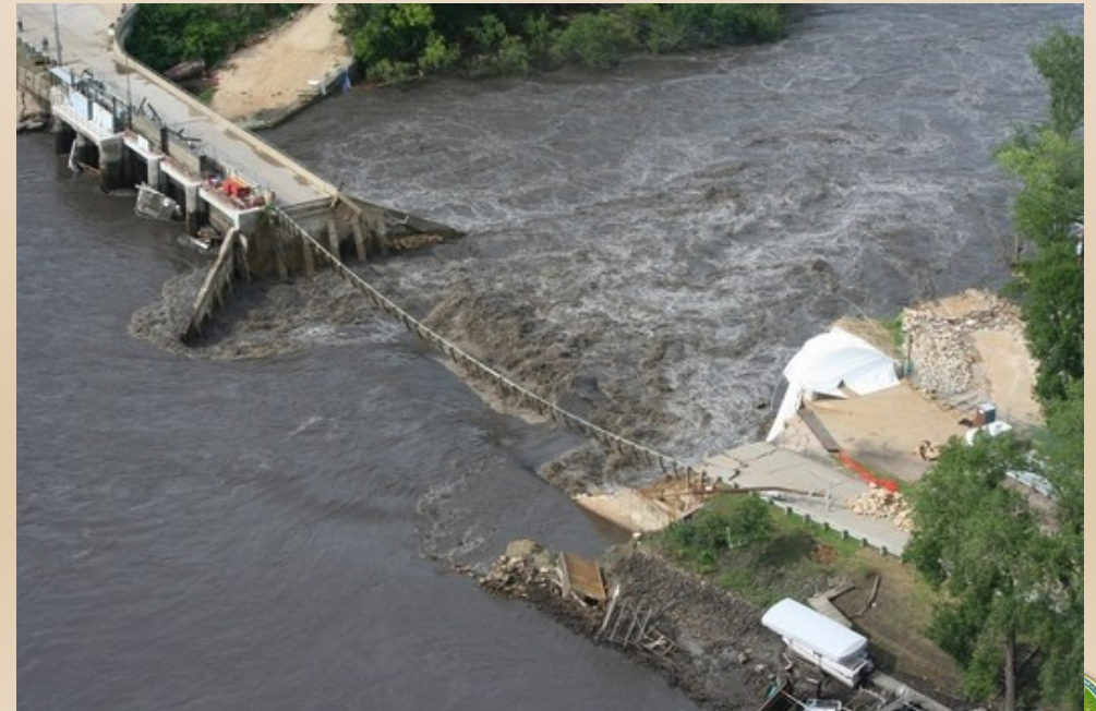
Lake Delhi Dam, Eastern Iowa July 24, 2010 Overtopping and Internal Erosion Failure (43 foot high embankment, 3,790 acre-ft)
