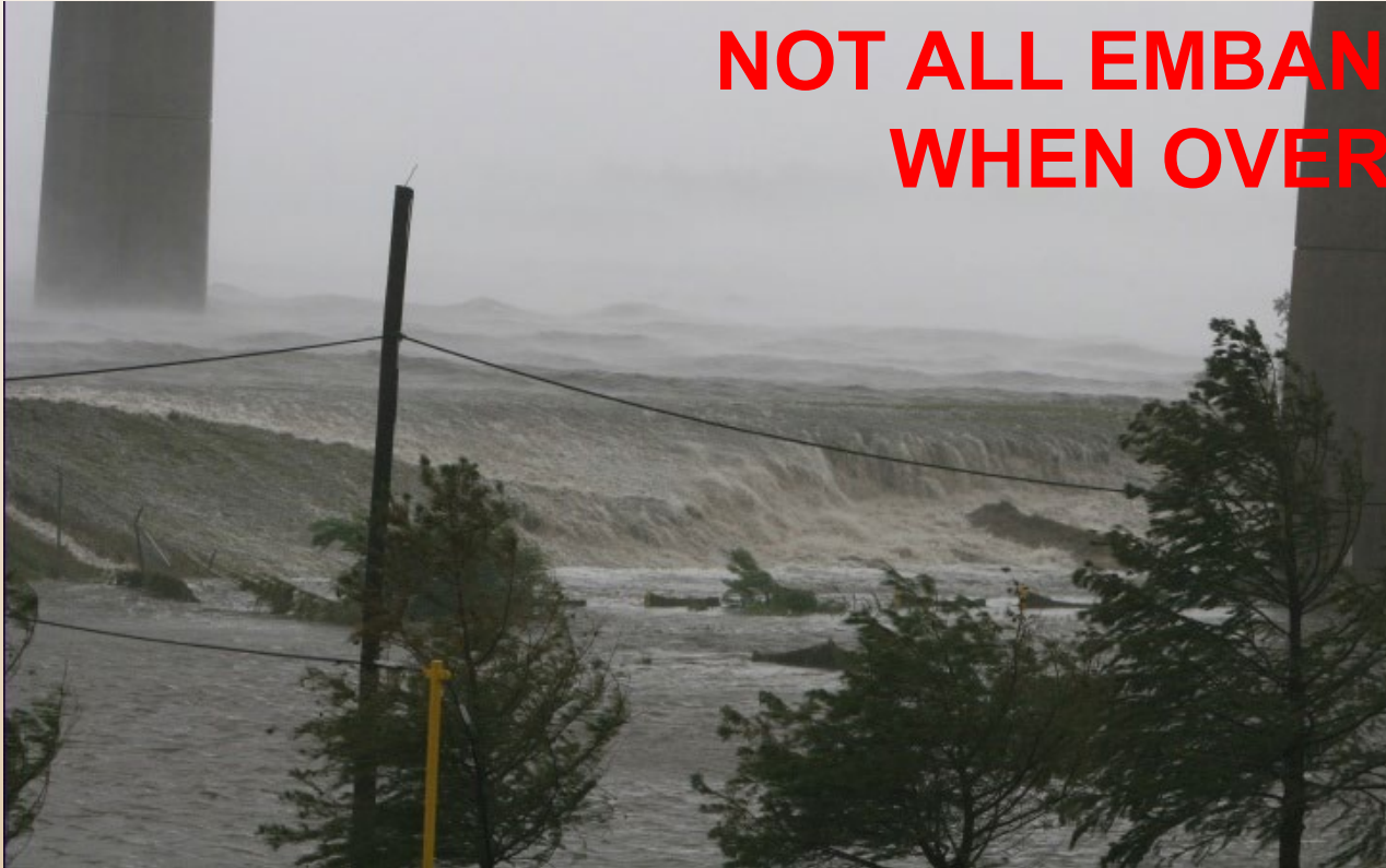
Levee on south alignment of New Orleans East at the Paris Road Bridge. Clay levee was overtopped but did not breach
