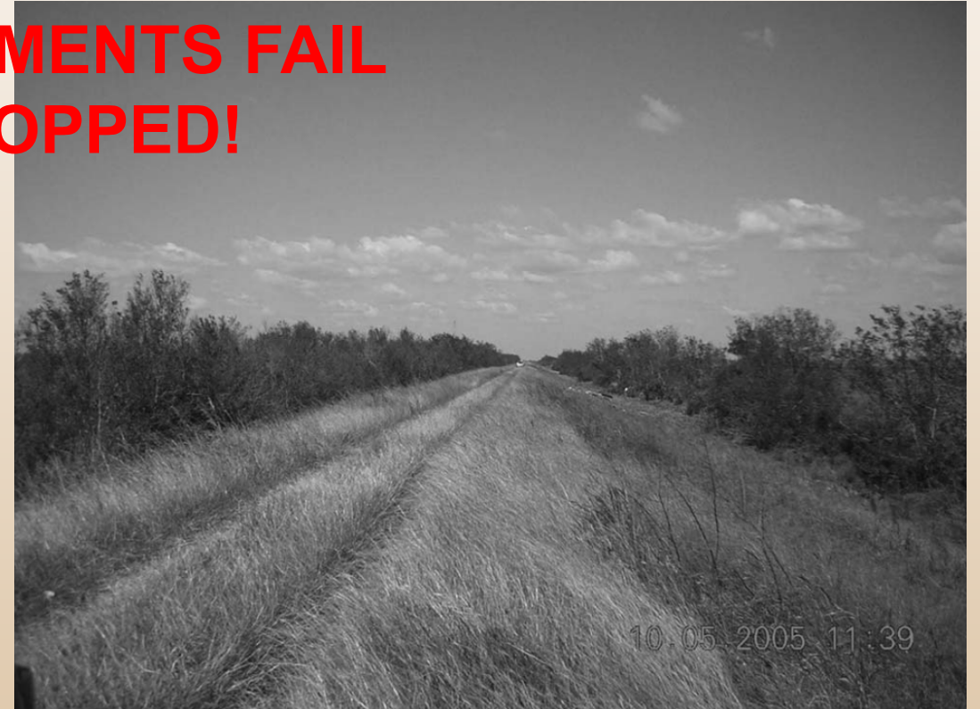
Levee section on the east edge of the New Orleans East protected basin showing a complete lack of erosional damage
