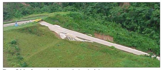
Figure F-2-9.—Overtopping along entire length of chute.
