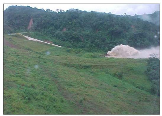
Figure F-2-8.—Sweepout of spillway stilling basin.
