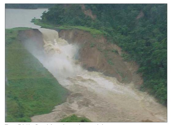
Figure F-2-12.—Breach formation nearing completion.
