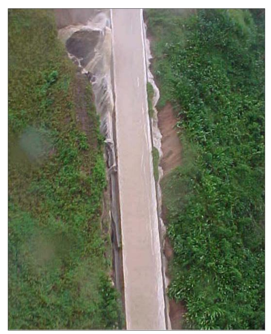
Figure F-2-10.—Overtopping of upstream chute walls.
