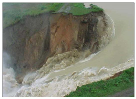
Figure F-2-11.—Headcutting progressed to reservoir.
