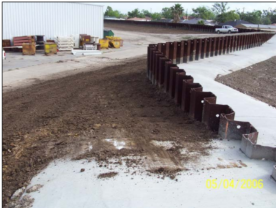
Figure E-8-6.—Overtopping scour protection for sheetpile I-wall.
