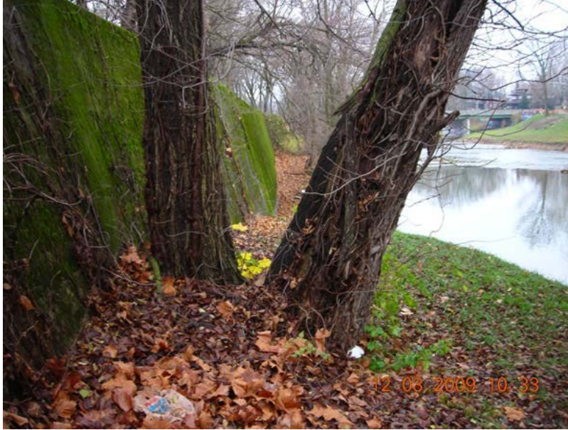
Figure E-8-7.—Large trees adjacent to floodwall.
