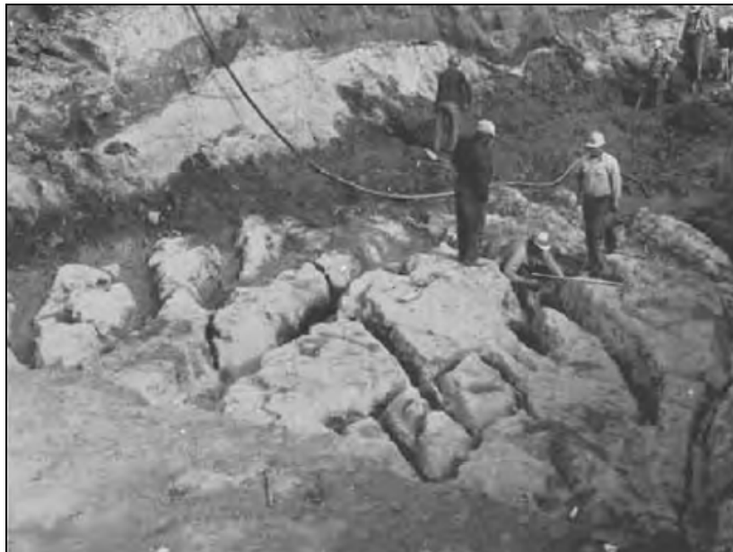
Figure A-4-5.—Typical limestone foundation joints.
