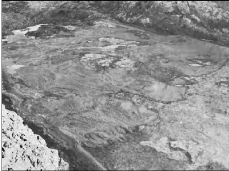
Figure A-4-6.—Rock foundation in cutoff trench after dental concrete treatment.
