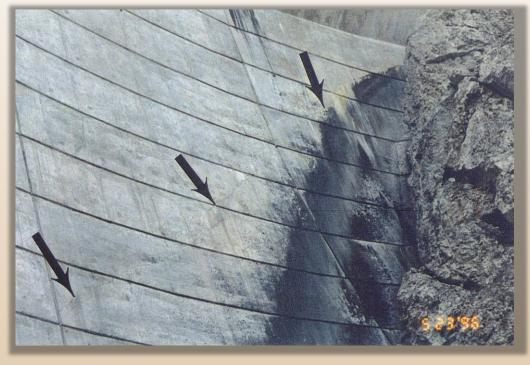
Cracks in **thin arch** dam from low reservoir and high temperature parallel to abutment. Upstream movement caused moment and tension on downstream face.
